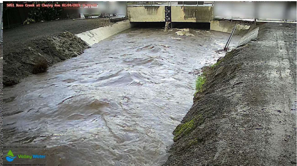
Cherry bridge 2-4-24 at 4 pm. 9 foot high bridge
