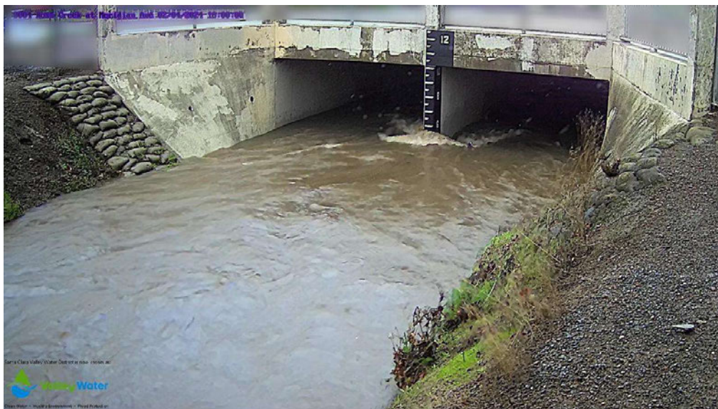
Meridian bridge 2-4-24 at 4 pm. 10 foot high bridge
