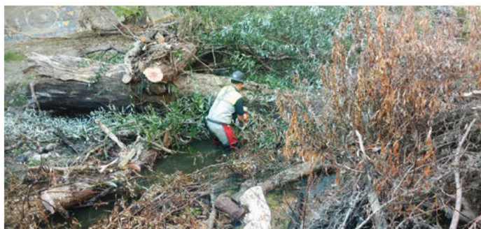
Staff removing fallen trees blocking creek flow.
