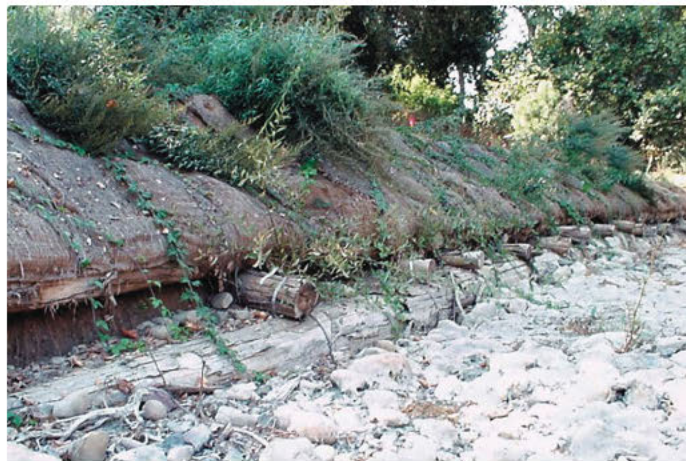
Site of completed erosion repair.
