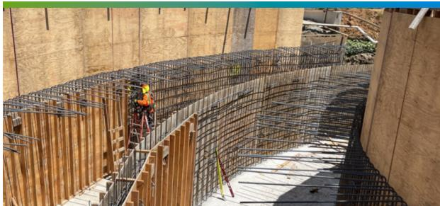
Crews built twin box culverts during the previous Phase 2A of the Upper Llagas Creek Flood Protection Project and will continue building these twin culverts along Hale Avenue towards Wright Avenue in Phase 2B.
