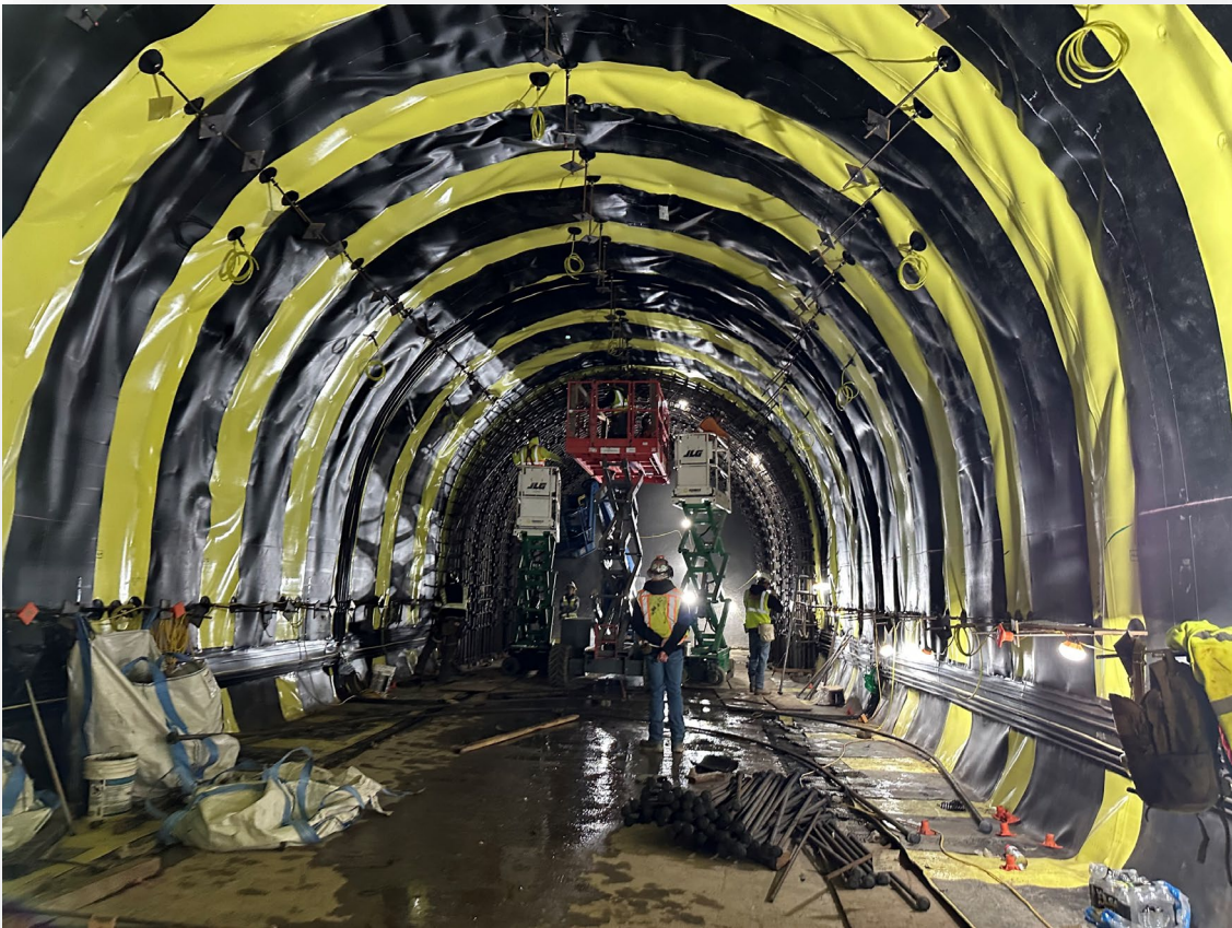
January 2025 Waterproof membrane inside the tunnel
