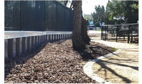
Vinyl sheet pile wall installed next to Rocksprings Park. The sheet pile will be replaced with longer and taller sheet pile wall.
