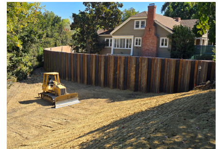
A floodwall was installed to protect homes along S. 17th Street and Coyote Creek.
