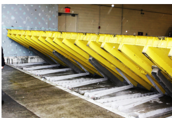
(top) A passive barrier installed in the closed position and embedded in the ground. (bottom) A passive barrier in the process of opening.
