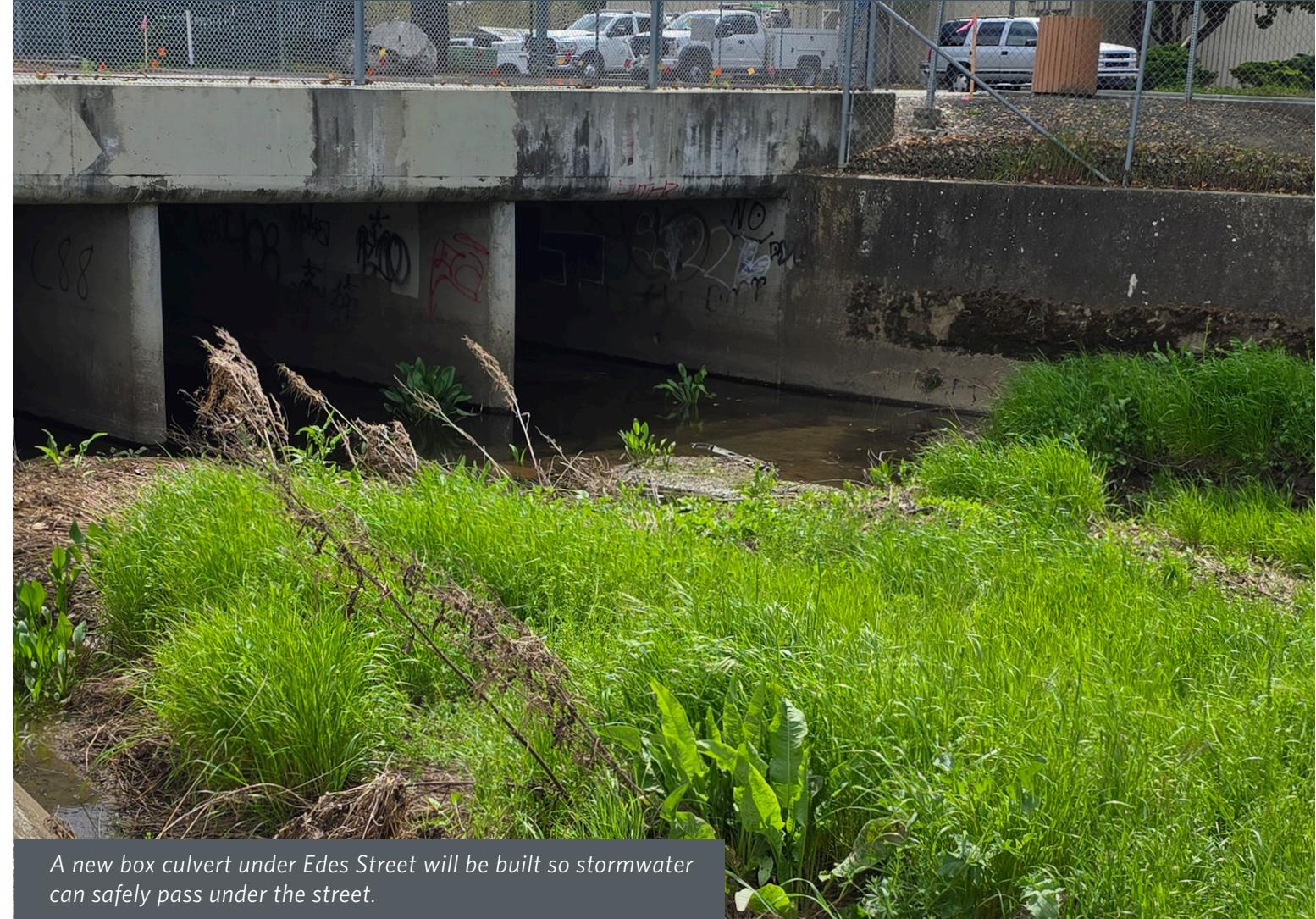
A new box culvert under Edes Street will be built so stormwater can safely pass under the street.
