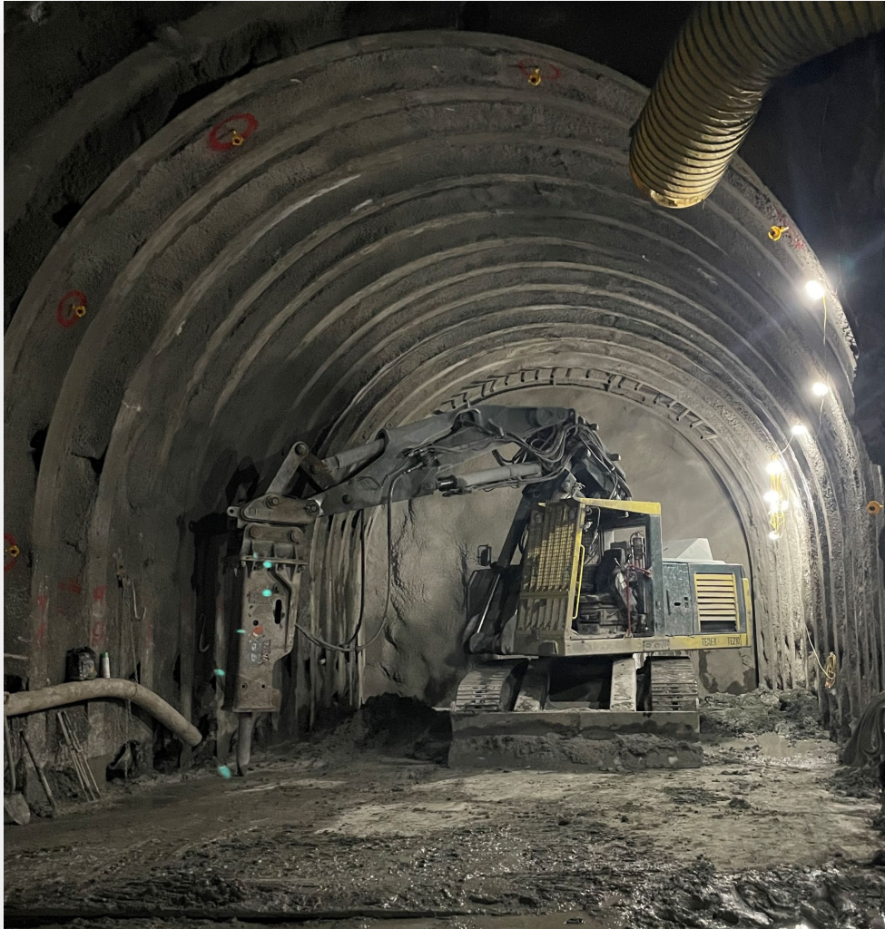
Excavator with hydraulic hammer
