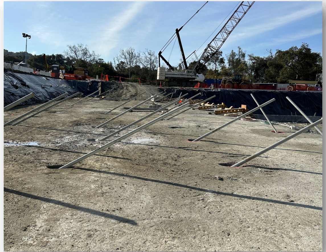
Rock Anchors installed through CLSM for DOS foundation
