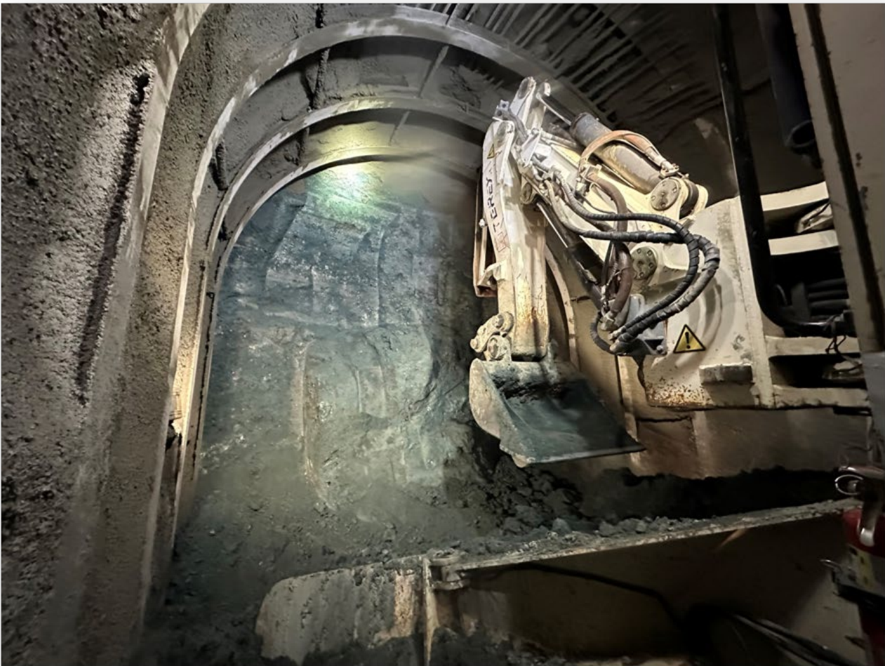
Tunnel excavation at face with bucket on the roadheader
