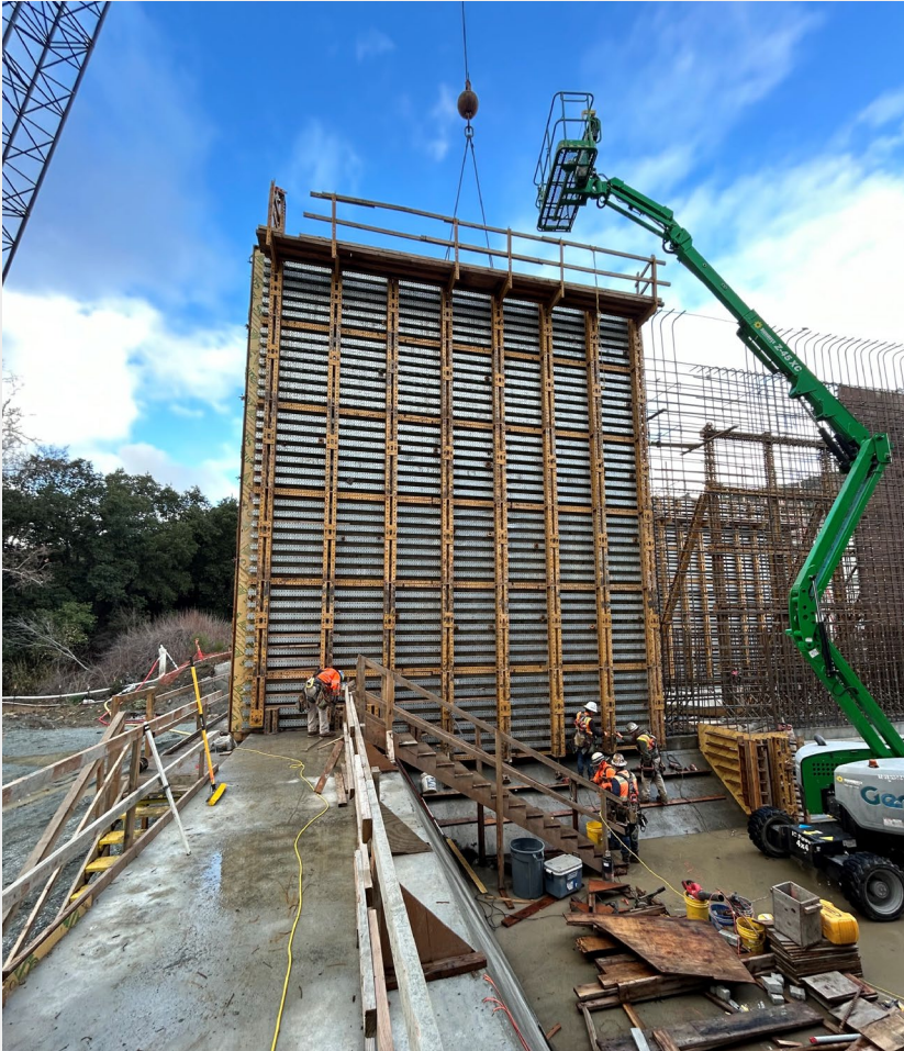
Middle wall formwork
