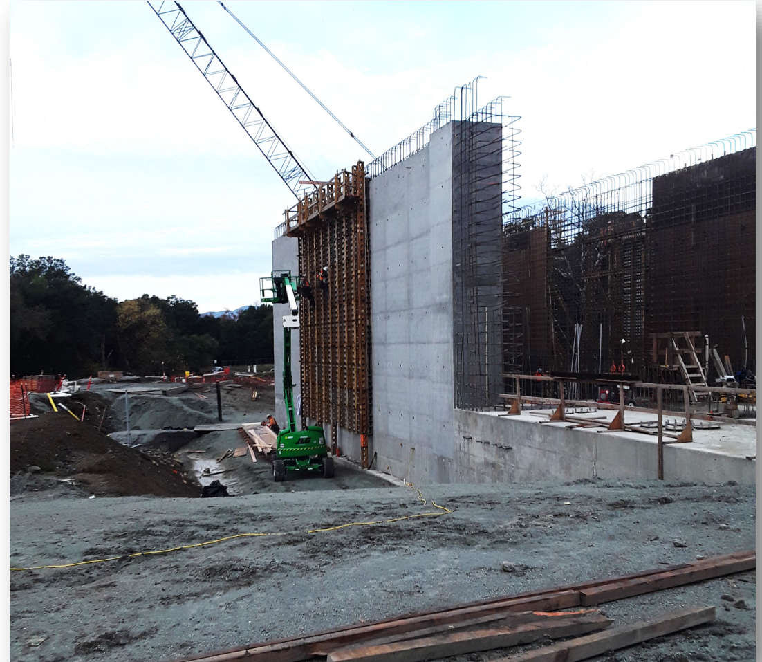
Outside wall formwork
