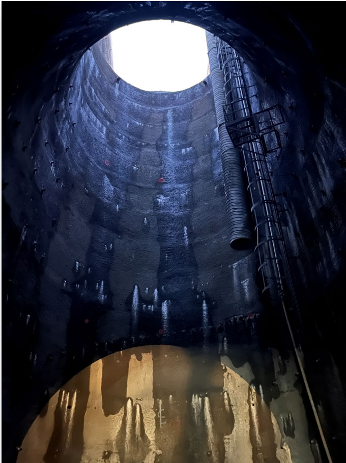
Completed Drop Shaft Excavation
