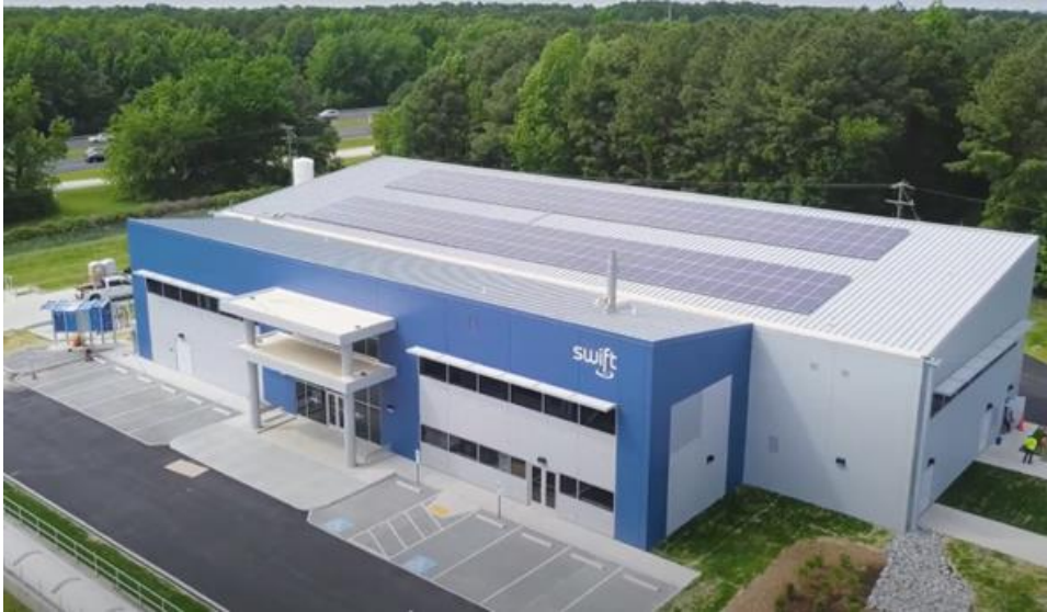
Figure 6: Hampton Roads Sanitation District Size: 1.0 MGD, Cost: $30M
