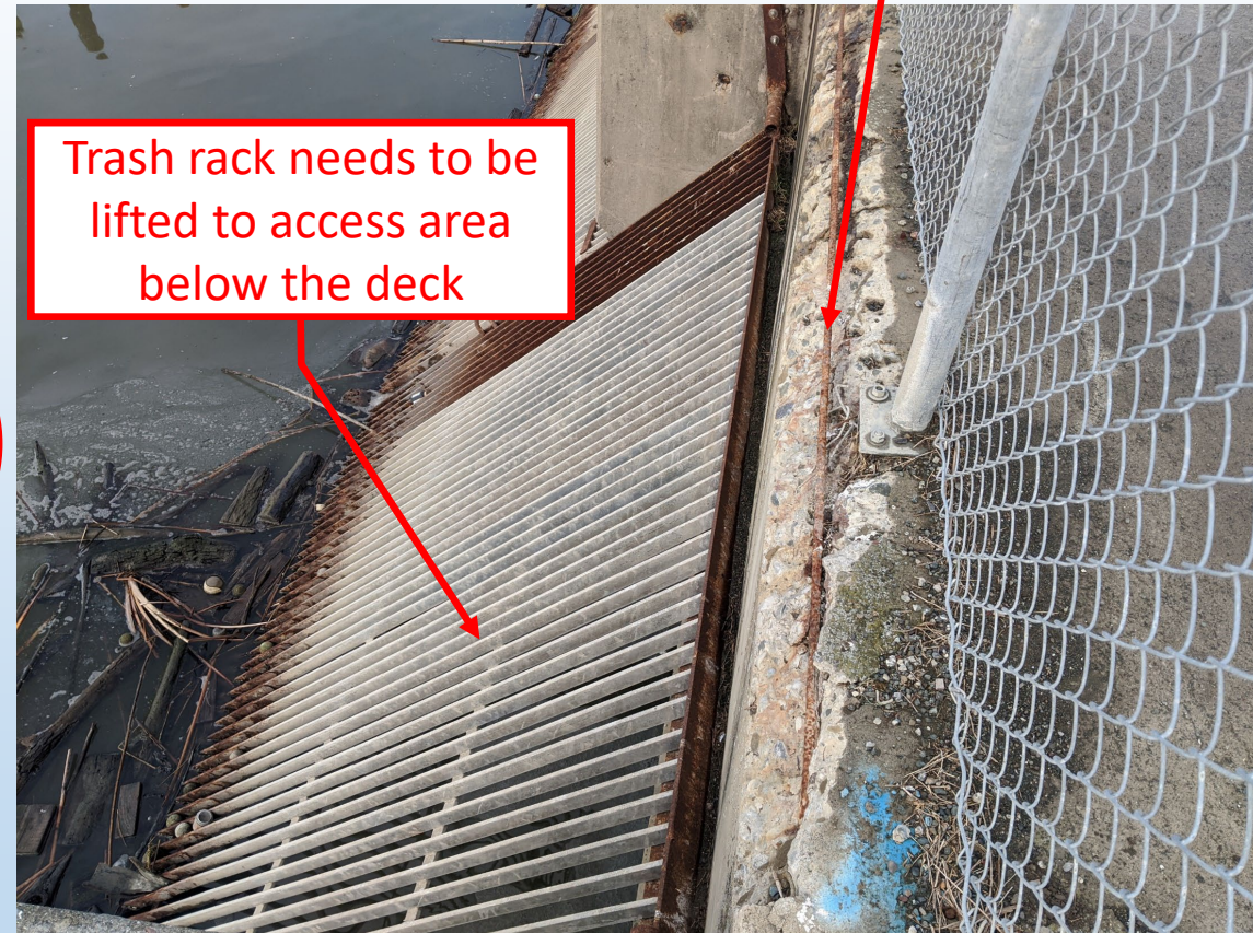
Trash rack located on the basin side.
