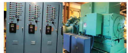
Existing Pump Control Panels (left) which will be replaced, and Pump Control Motors (right) which will be rehabilitated as part of the Coyote Pumping Plant Adjustable Speed Drive Replacement Project.
