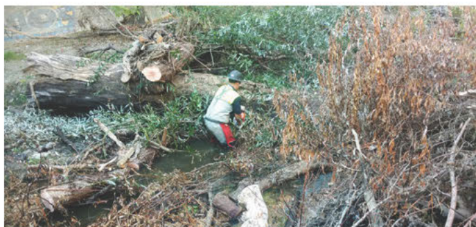
Staff removing fallen trees blocking creek flow.
