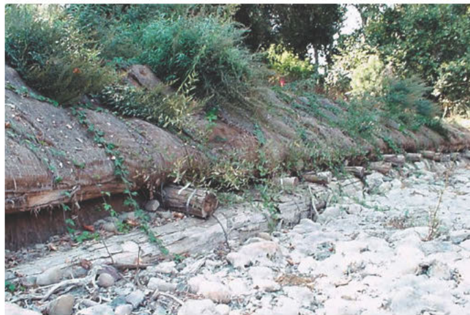
Site of completed erosion repair.
