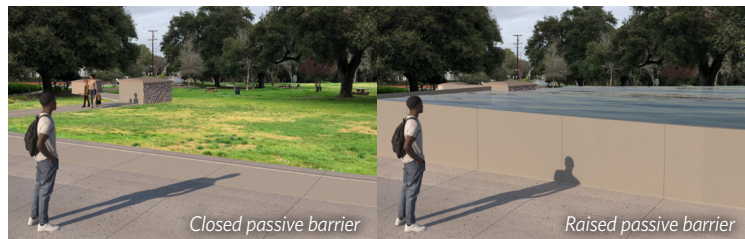
At Williams Street Park, located along South 16th Street, there are plans for a passive barrier that once completed, will retain floodwater in the park and prevent it from entering the surrounding neighborhood.
