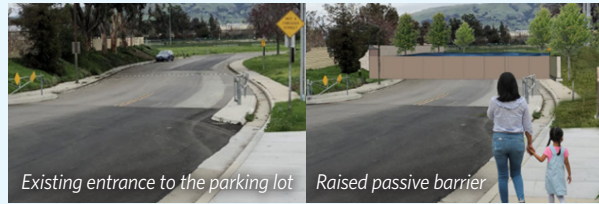
Existing entrance to the parking lot Raised passive barrier A flood barrier will be installed at the Jackson Street parking lot entrance.
