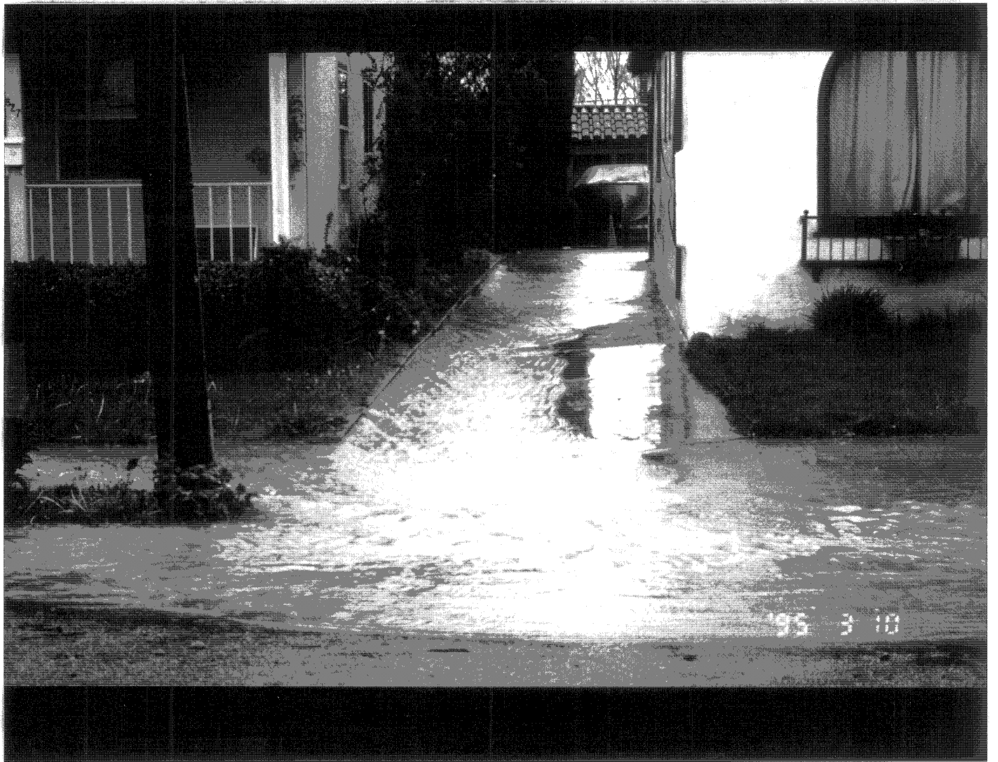
FLOODING FROM GUADALUPE RIVER AT HARLISS AVE. 3/10/95 112
