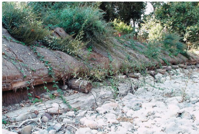
Site of completed erosion repair.
