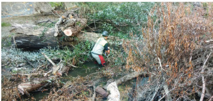
Staff removing fallen trees blocking creek flow.
