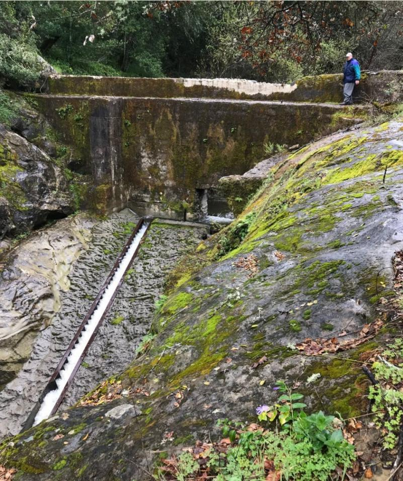
**After** – Removal of the > 100 year old dam will enable access to ~3.5miles of high-quality spawning and rearing habitat for steelhead and will allow the stream to return to its natural processes, facilitating natural instream habitat feature formation.
