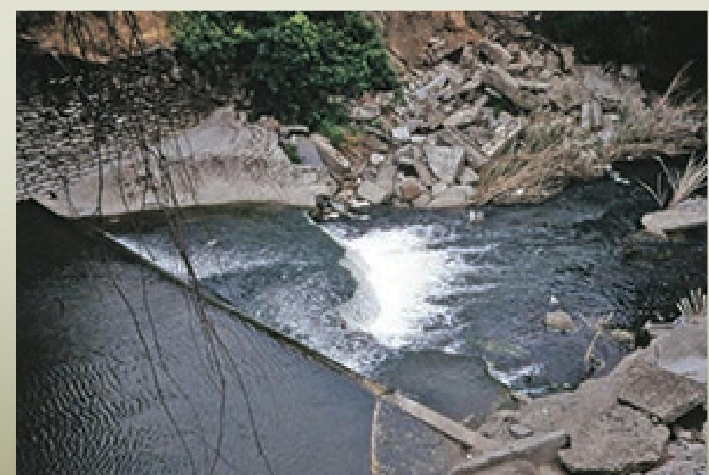
**Before-** The concrete apron associated with the Hillsdale Bridge and deteriorated stream conditions downstream were impeding fish passage
