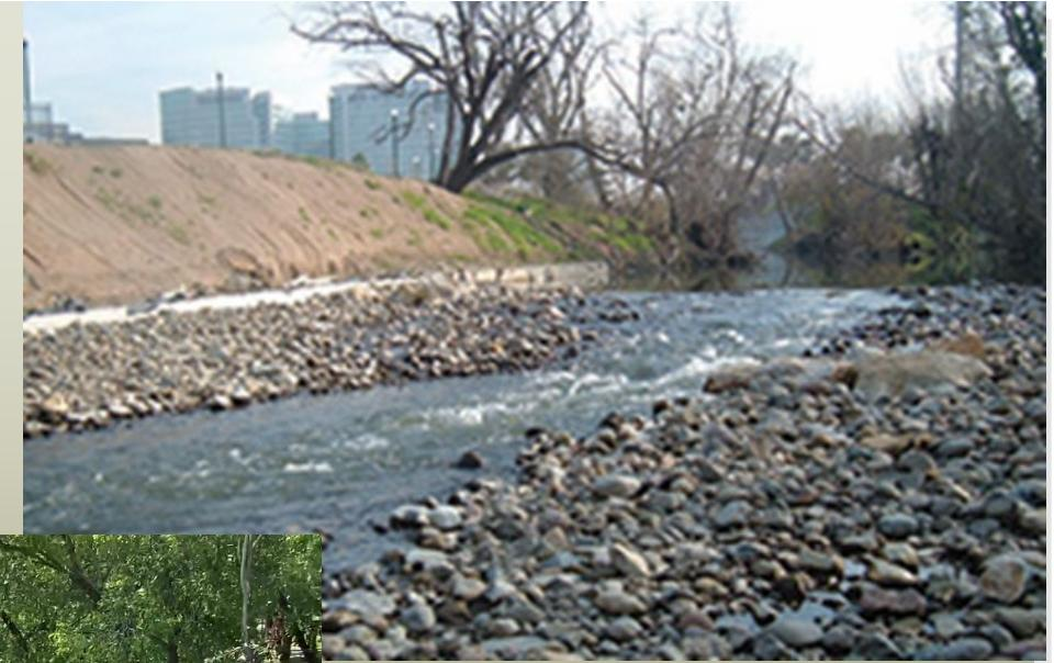
**After-** Replaced the existing weir with stepped riffles that provided habitat, enhanced fish passage and improved channel stability.
