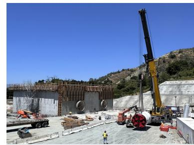
Diversion Outlet Structure nearly complete. Micro Tunnel Boring Machine assembly.
