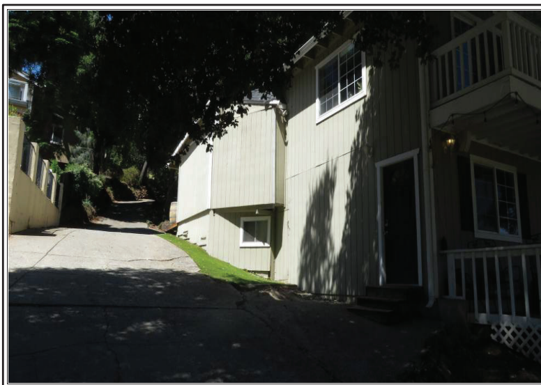
SUBJECT'S SOUTH SIDE
