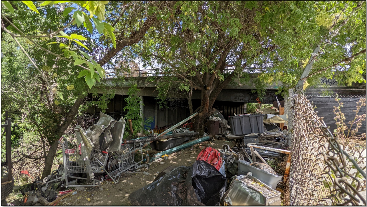
View of PE 295 and TCE 378 located near the street frontage, as seen from northeast portion of the subject site looking towards Berryessa Road
