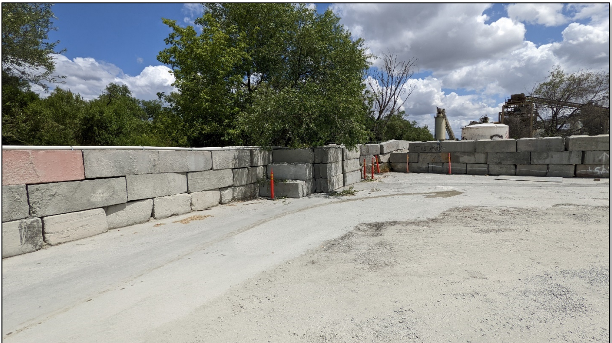
View of TCE 379 located on the rear parcel, facing southeast
