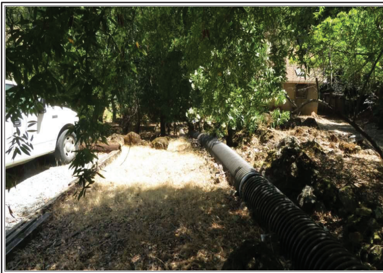
SUBJECT'S WEST BOUNDARY LOOKING EAST/DRAINAGE PIPE
