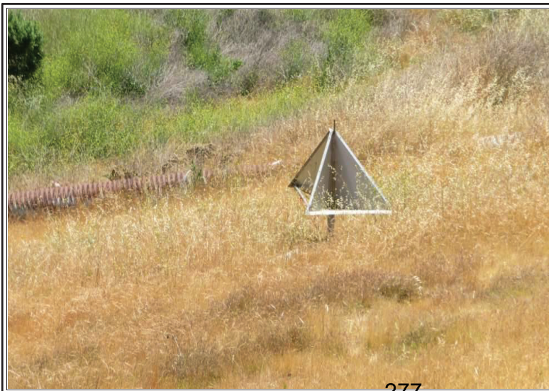
SUBJECT'S SEISMIC DETECTOR
