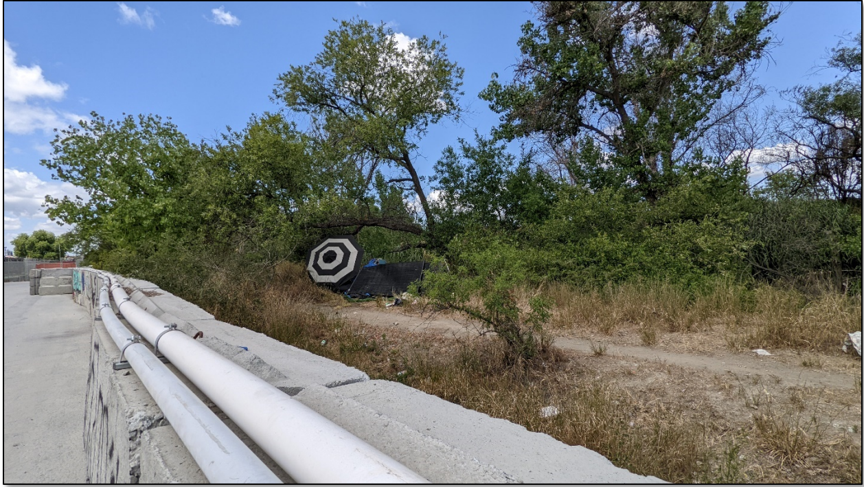
View of PE 296 and TCE 379 on the rear parcel, as seen from the subject's northeastern lot line facing northwest
