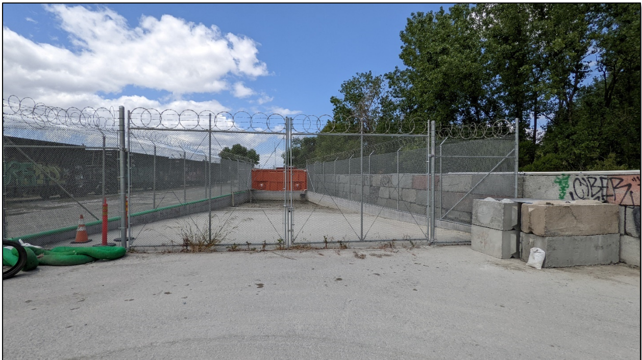
View of the improvements associated with the on-site storm drainage system that are impacted
