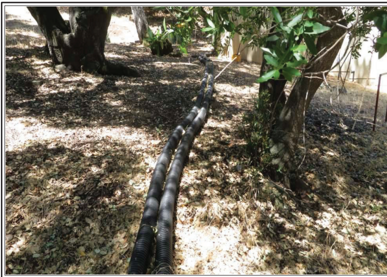
REAR OF SUBJECT PROPERTY LOOKING SOUTH
