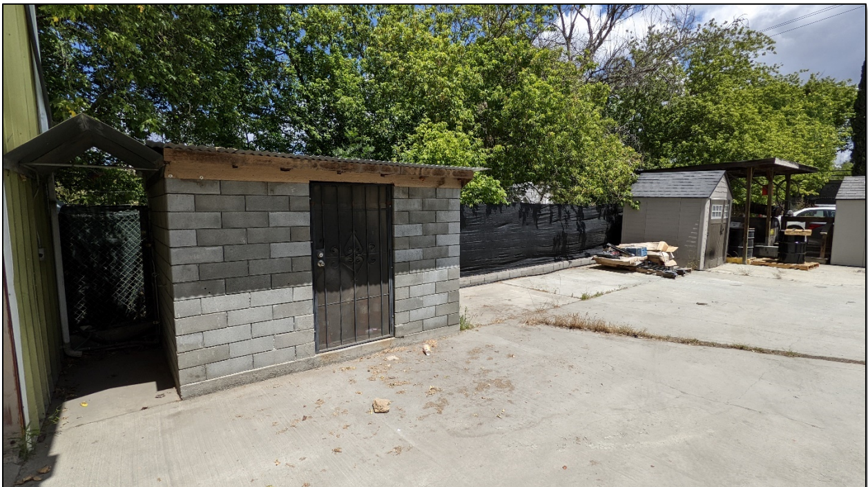
View of the TCE 378 located to the east of the utility building
