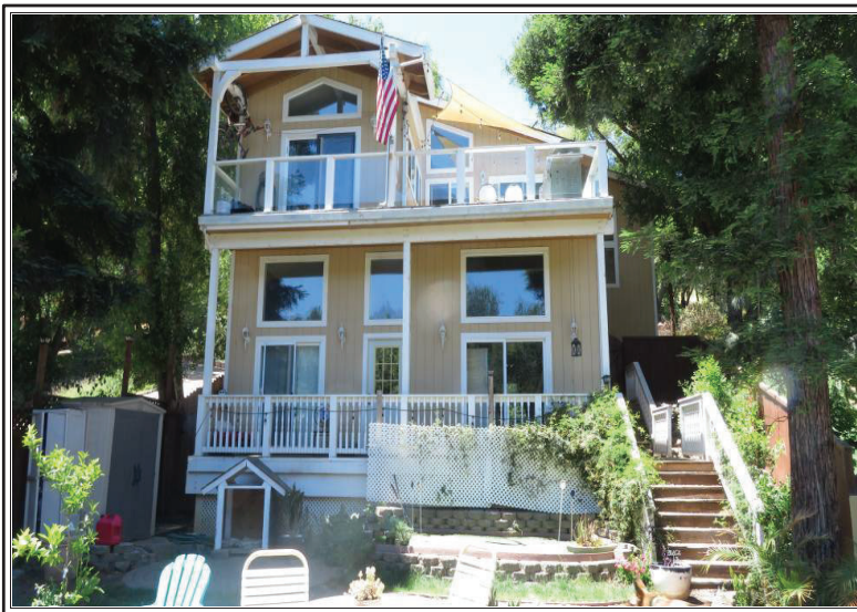
REAR OF SUBJECT PROPERTY
