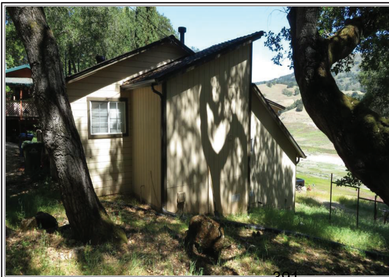
SUBJECT'S SOUTHERN SIDE
