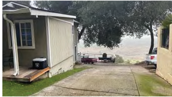
Right: Concrete driveway extending to lakebed – driveway is shared with property adjacent to the south
