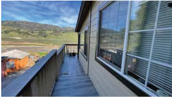
Left: Deck Right: Deck on northerly side of residence
