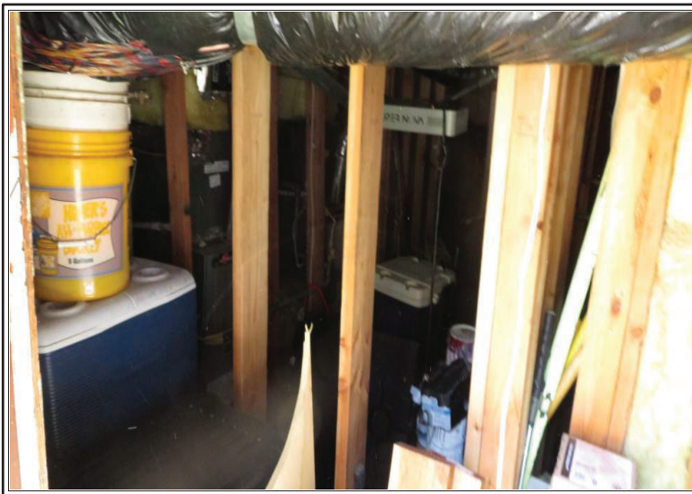
SUBJECT'S STORAGE AREA LOWER LEVEL
