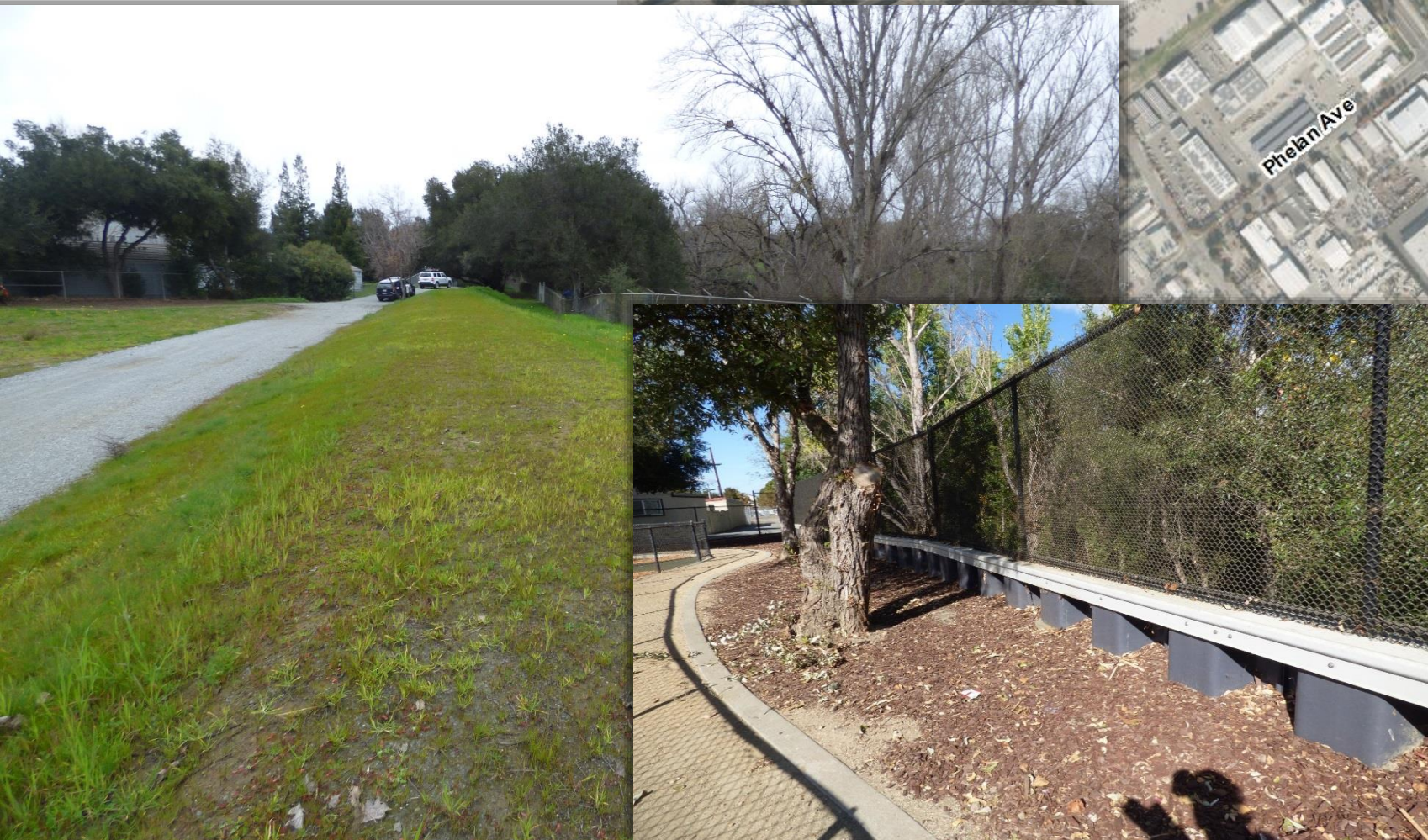
Figure 4.32. Existing berm and floodwall at Rock Springs neighborhood. Location of proposed berm and floodwall in the area is similar to existing. Proposed floodwall and berm would be about 1.5-ft taller than existing.
