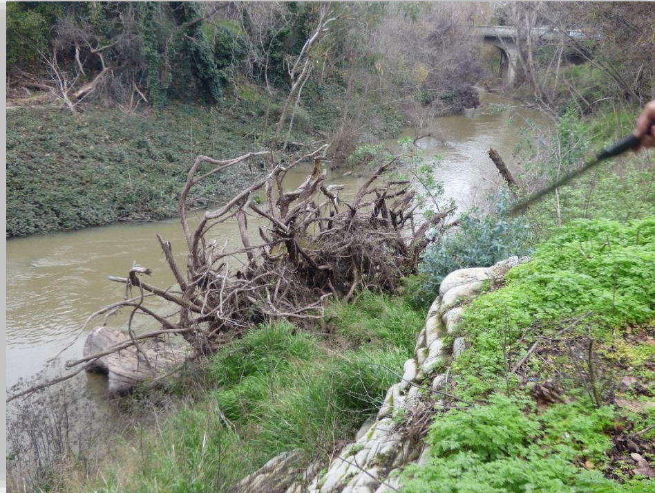
Figure 3.40. East bank Coyote Creek, south of East Julian Street, sacked concrete observed to halt evidence of erosion on the area
