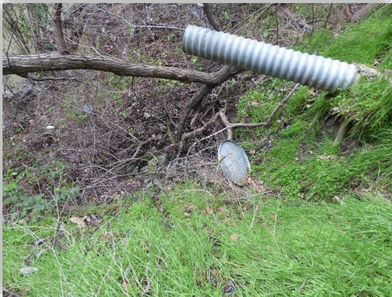
Figure 3.38. East bank Coyote Creek, north of East Julian Street, exposed storm drain outfall and observed erosion
