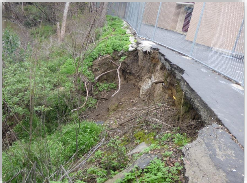
Figure 3.39. East bank Coyote Creek, south of East Julian Street, exposed storm drain outfall and observed erosion
