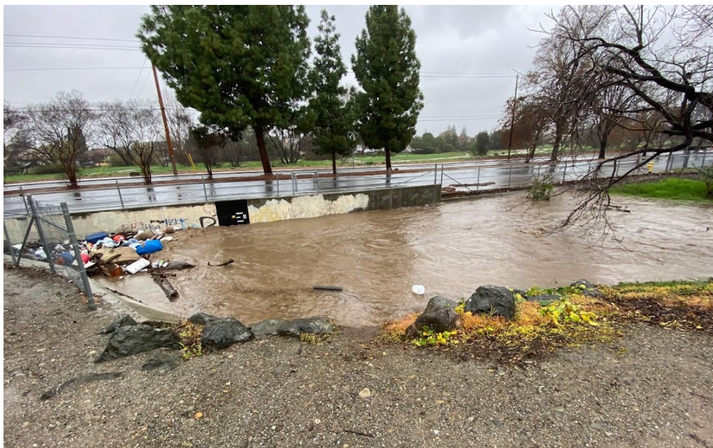
Figure 15. Upper Penitencia Creek at Mabury Road near Pine Hollow Circle (12/31/22)
