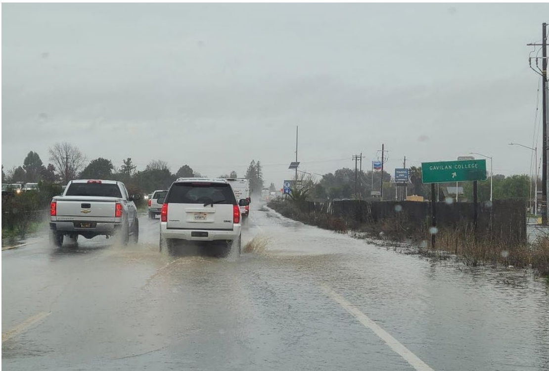
Figure 29. Uvas Creek Overbanking Flooding US-101 (1/9/23)
