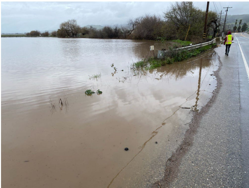
Figure 45. Flooding from Jones Creek upstream of Pacheco Pass Hwy, looking east (1/14/23)
