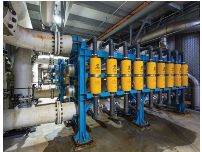
Energy recover devices used to capture hydraulic energy at the Carlsbad Desalination Plant.
