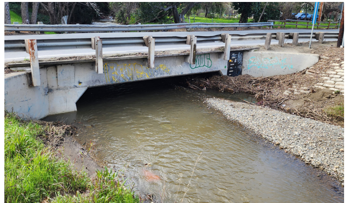
Upper Penitencia Creek will be redesigned to allow more stormwater to pass safely under the City of San José's King Road bridge.
