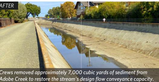
*Crews removed approximately 7,000 cubic yards of sediment from Adobe Creek to restore the stream's design flow conveyance capacity.*
