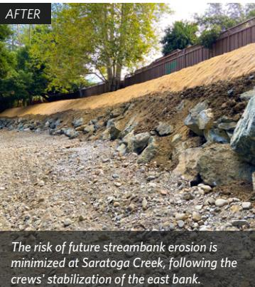
*The risk of future streambank erosion is minimized at Saratoga Creek, following the crews' stabilization of the east bank.*
