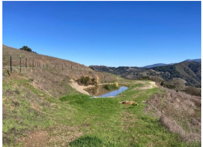
After its restoration, Pond RC-07 can securely hold rainwater.
