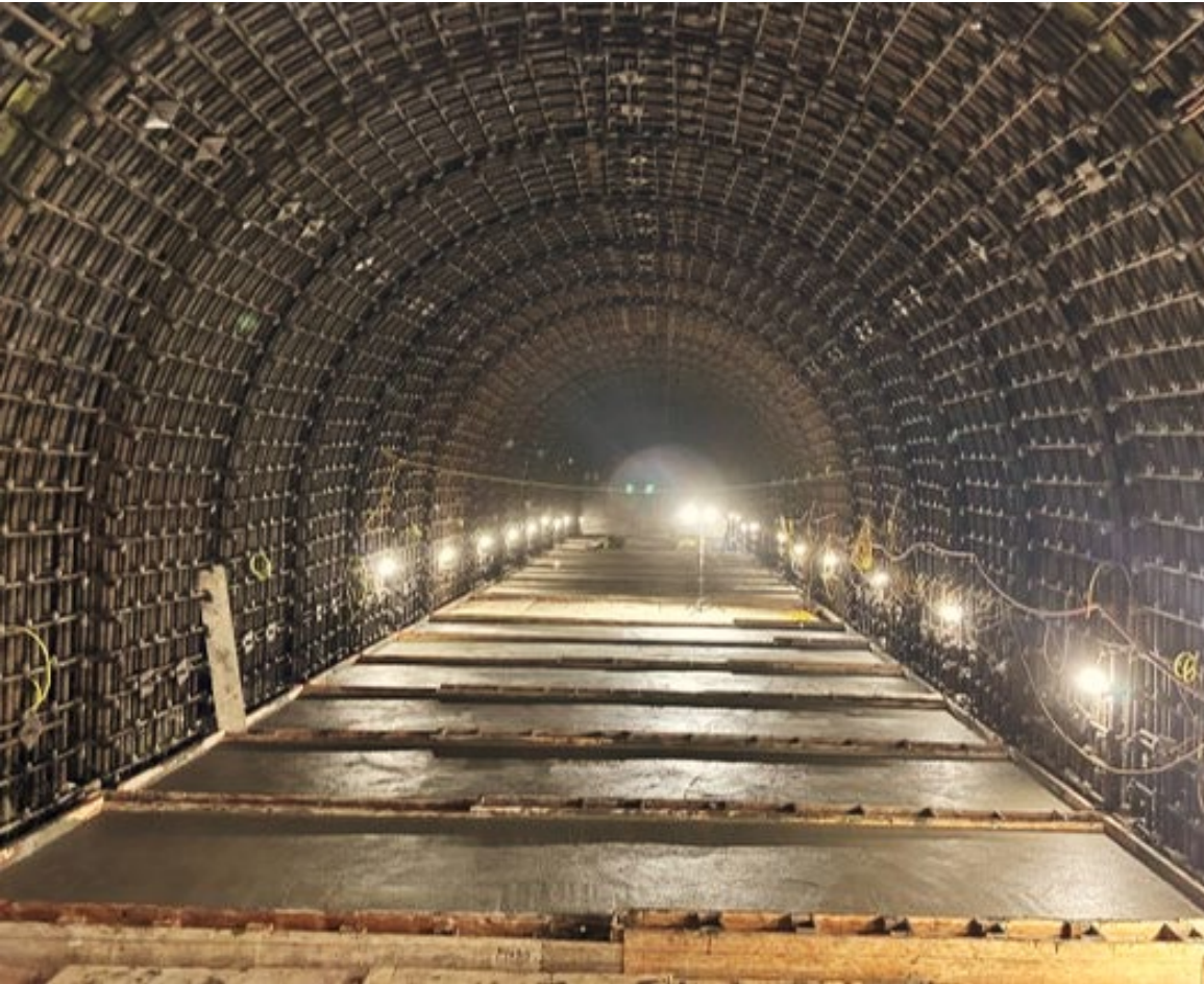
September 2025 Upstream Segment - Placed concrete for invert floor.
