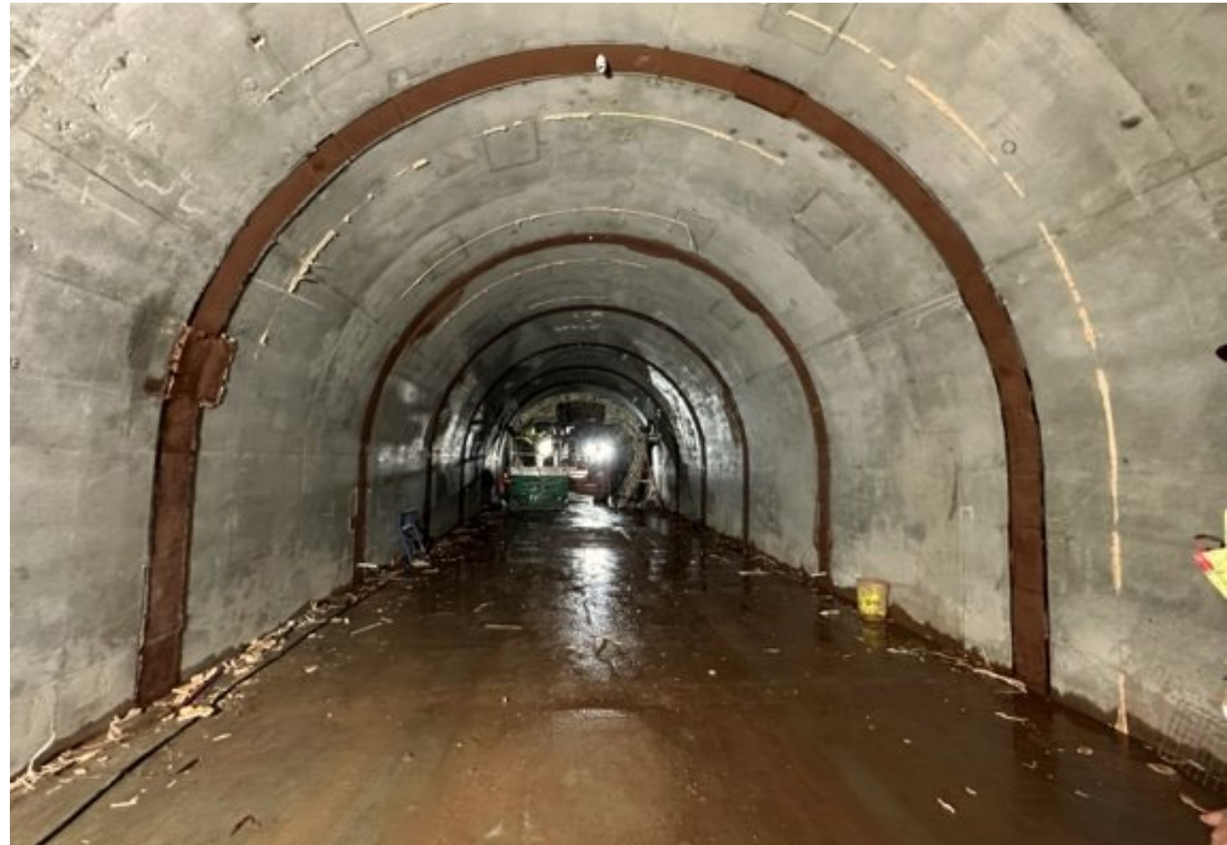
February 2026 Upstream Segment – Concrete placement for walls, arches, and gaps.
