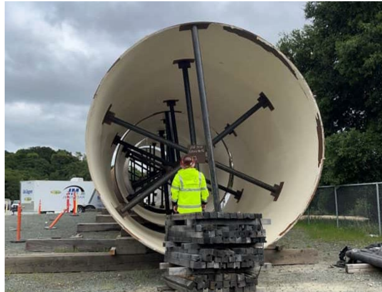
April 2025 Sections of 13-foot diameter steel pipes on site.
