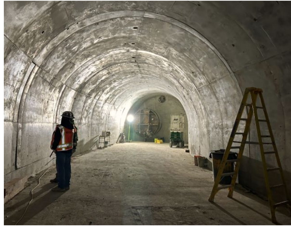
February 2026 Completion of the concrete final lining
