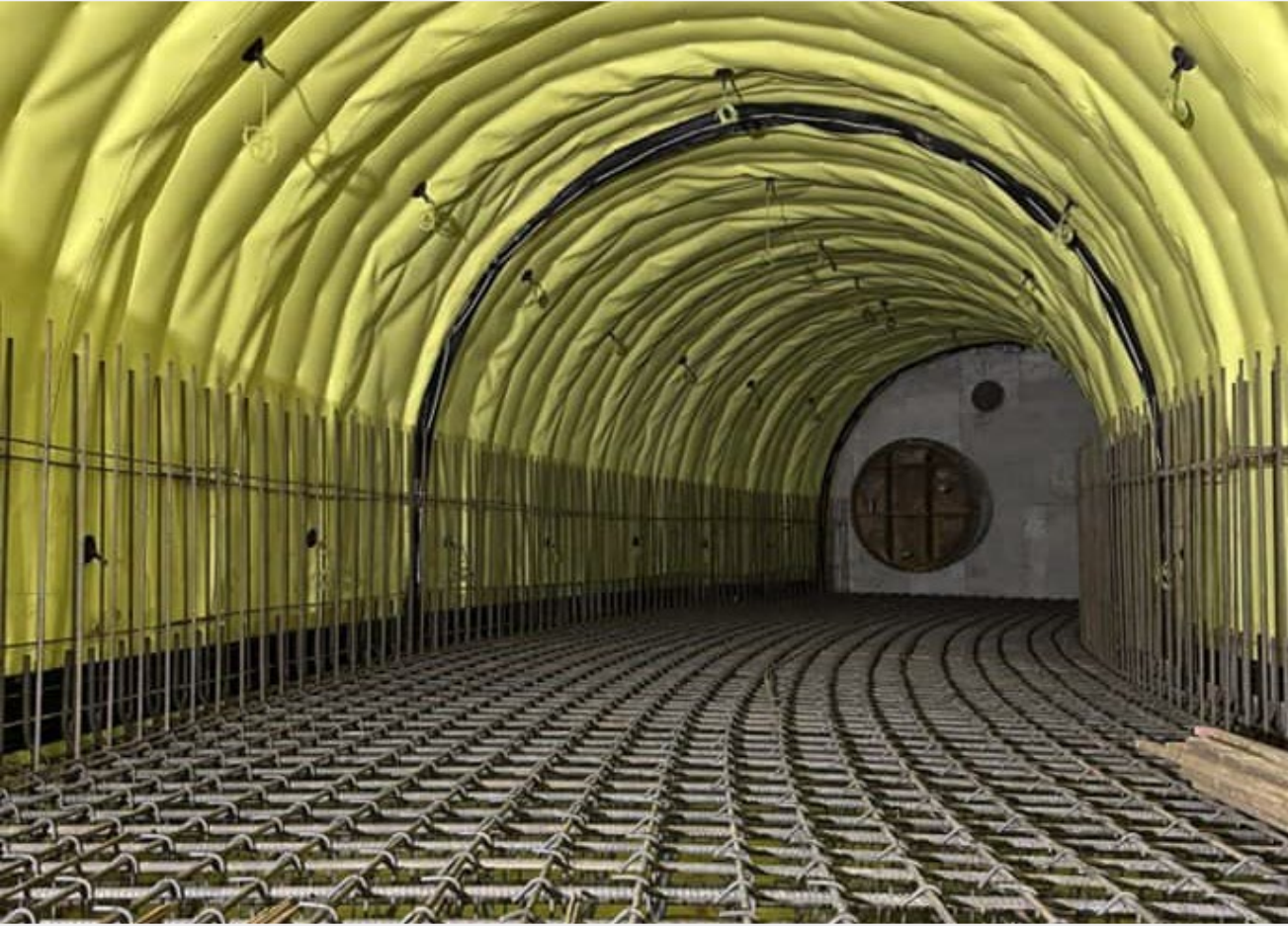
September 2025 Tunnel waterproofing and invert rebar in place.
