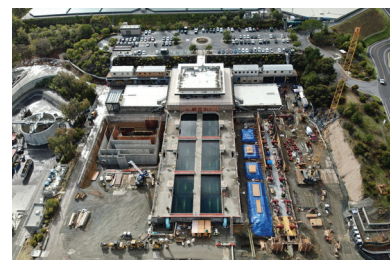
Phase 4 construction progress of Rinconada Reliability Improvement Project.
