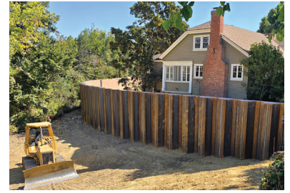
A floodwall behind a home on South 17th Street.
