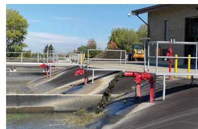
Sludge Pond Filling
