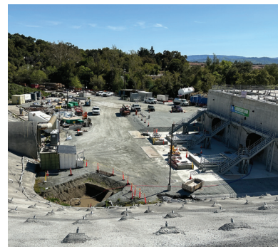
Nearly completed construction of the Anderson Outlet Tunnel.
