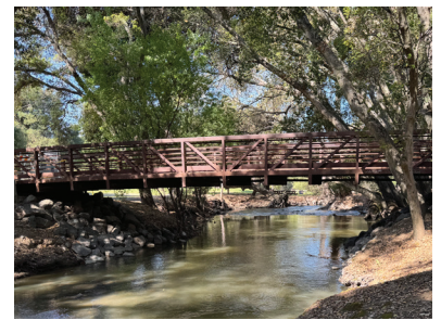
Pedestrian Bridge at Live Oak along Coyote Creek.
