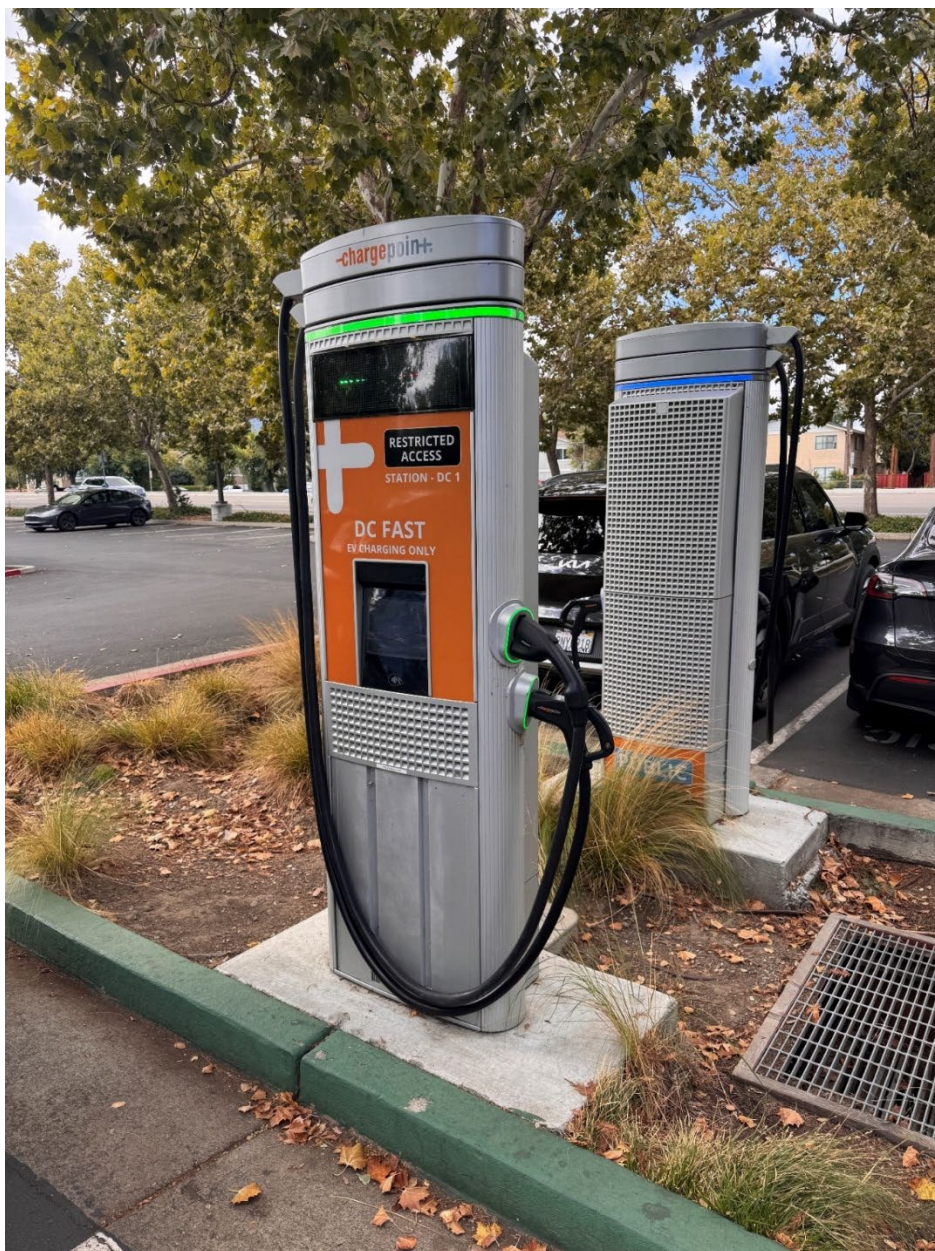
Figure 2-11. Existing Level 3 EV Charger
