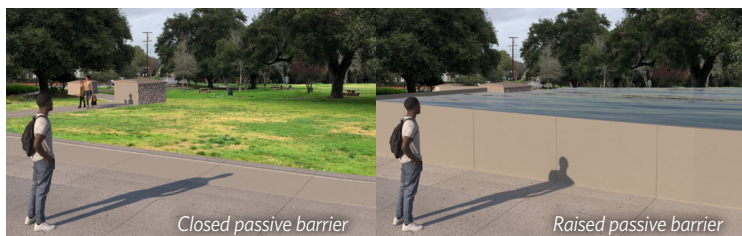
At William Street Park, located along South 16th Street, there are plans for a passive barrier that once completed, will retain floodwater in the park and prevent it from entering the surrounding neighborhood.
