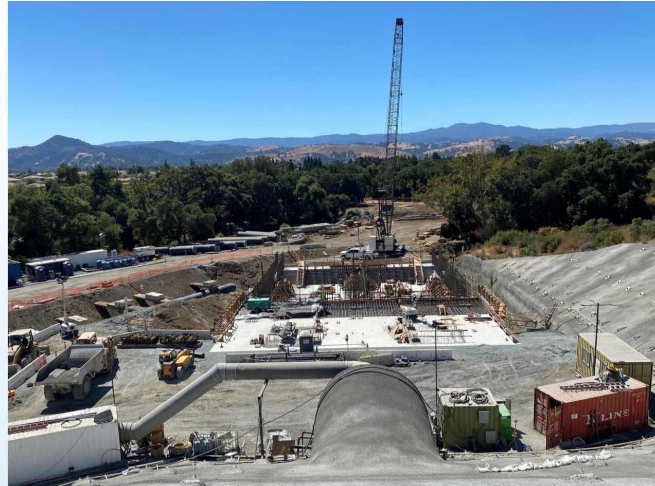
Diversion Outlet Structure construction September 2023
