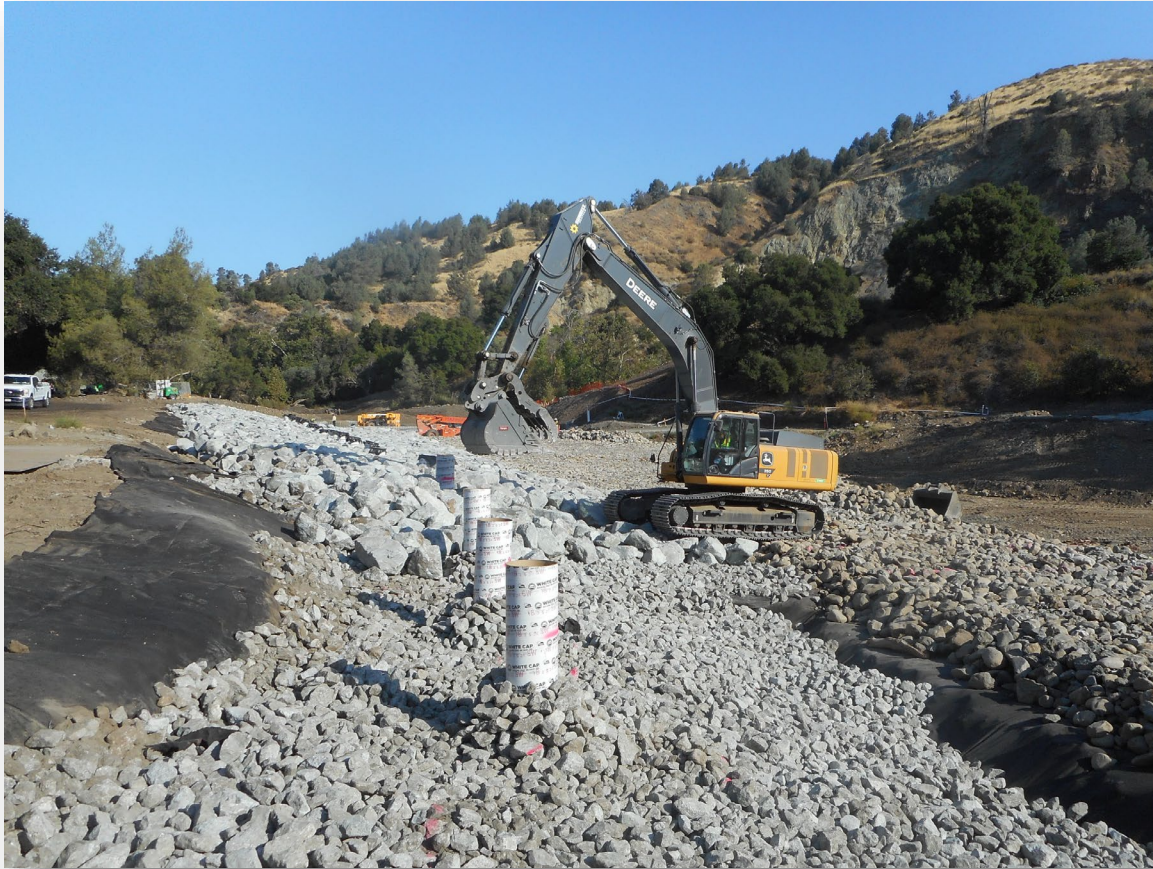
July 2024 Placing rock in the North Channel
