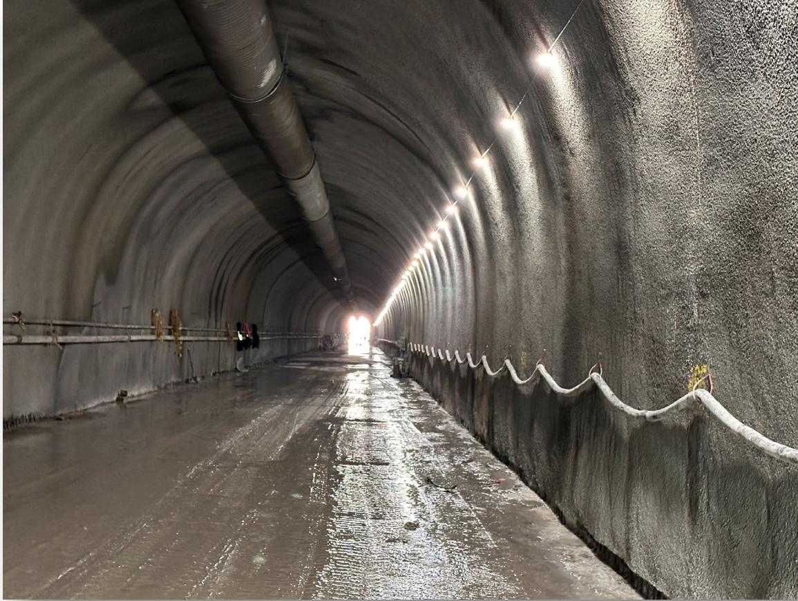
April 2024 Completed tunnel excavation and initial lining
