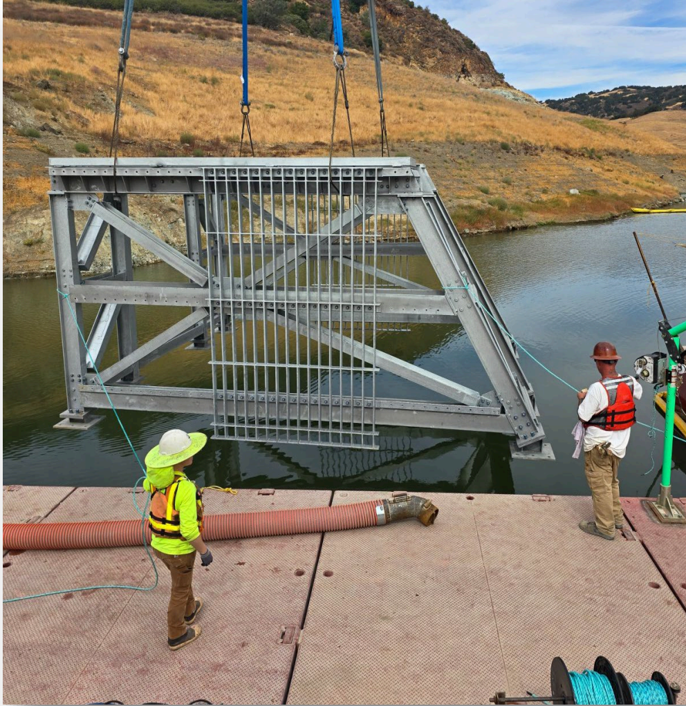
Lake Tap intake trash rack
