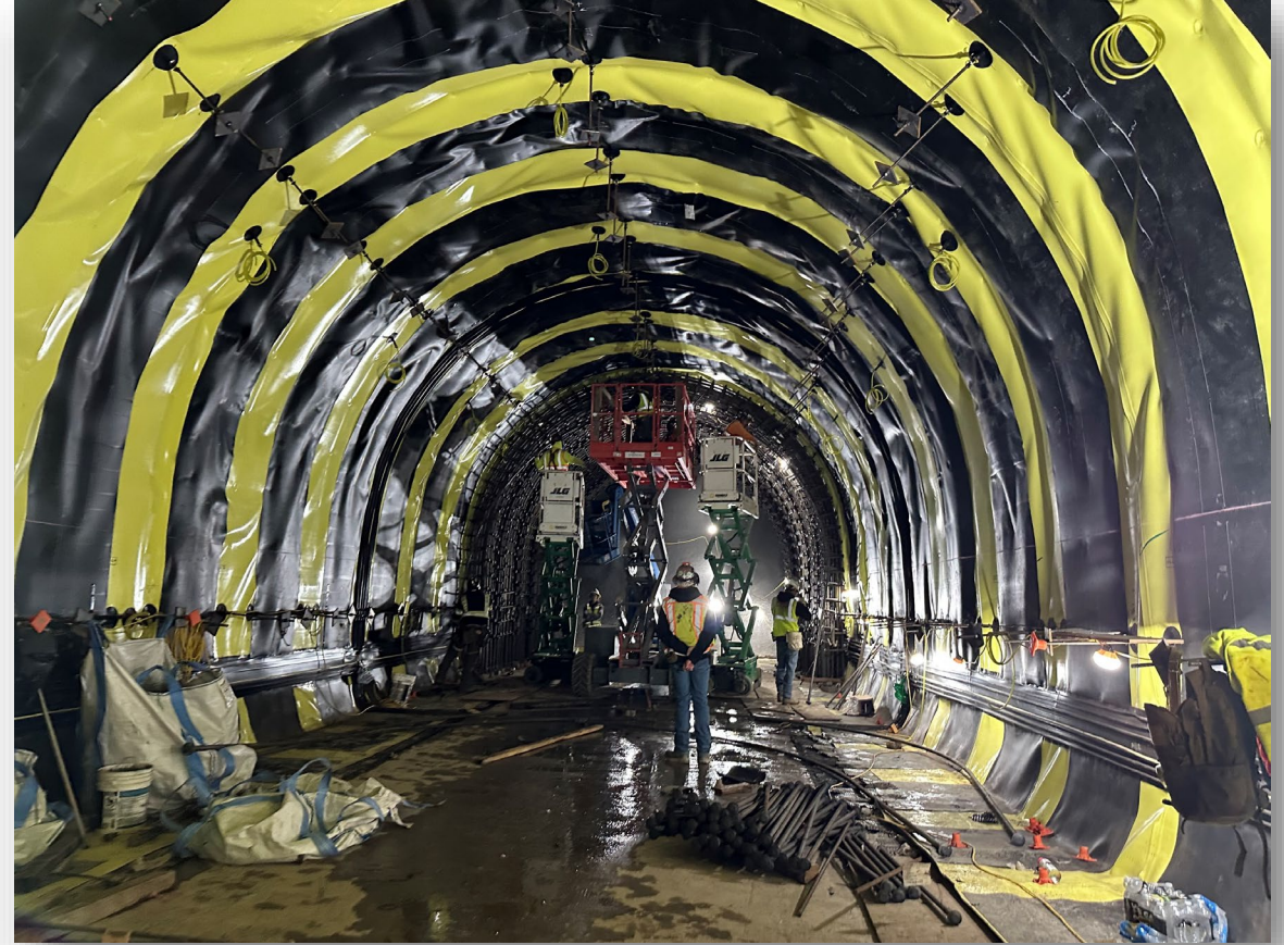
January 2025 Waterproof membrane inside the tunnel
