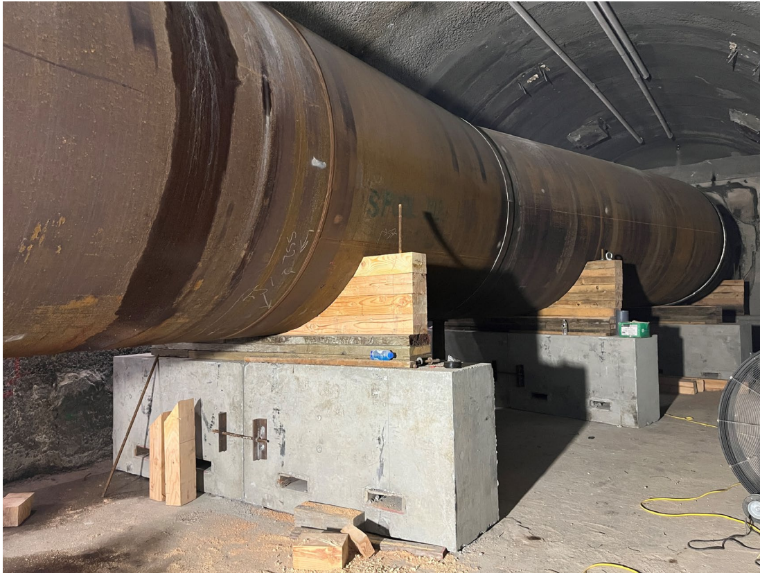
April 2025 8-foot diameter pipe extension with precast saddles
