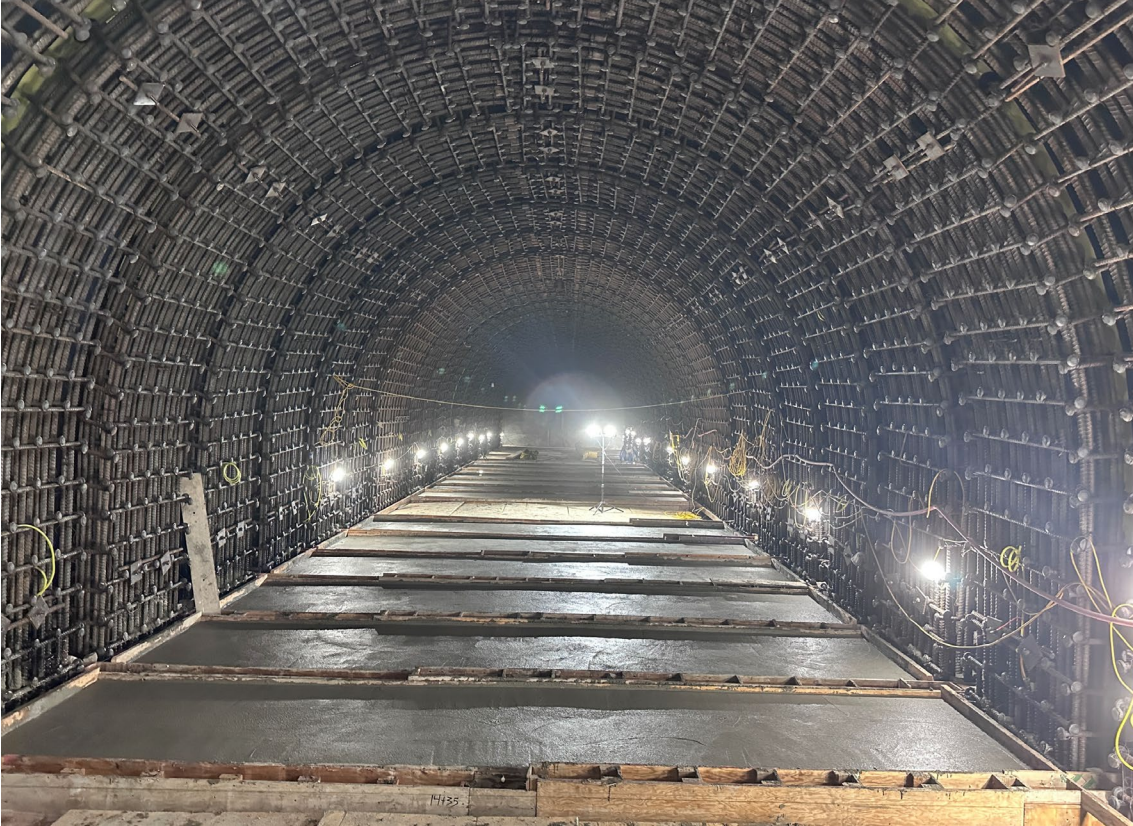
Upstream Leg - invert (floor) concrete placed
