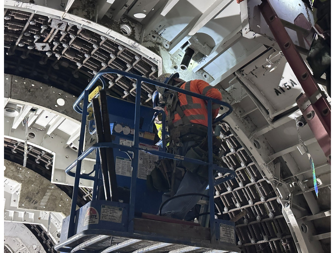
Downstream Leg - formwork installation for the arch concrete
