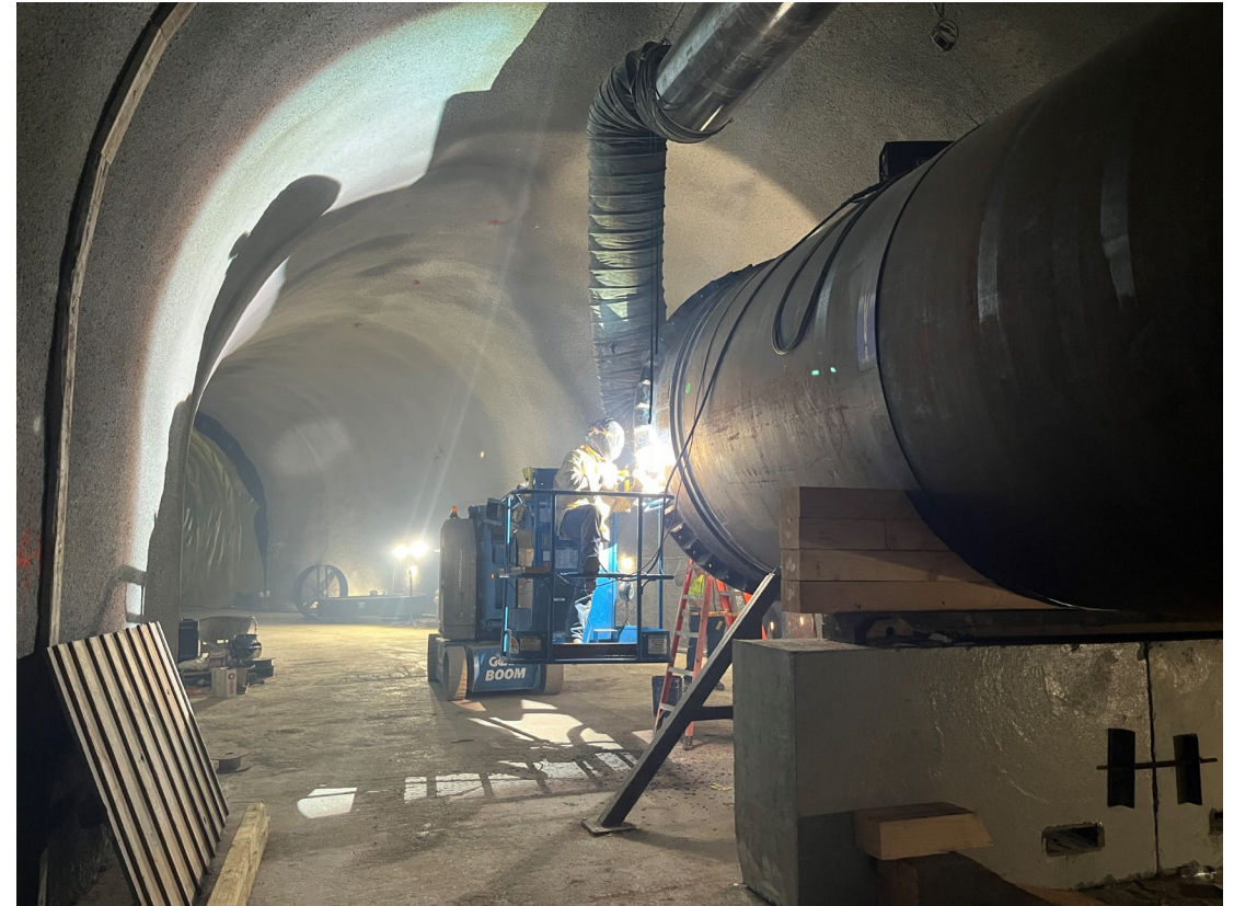
April 2025 Completion of the 8-foot diameter pipe extension
