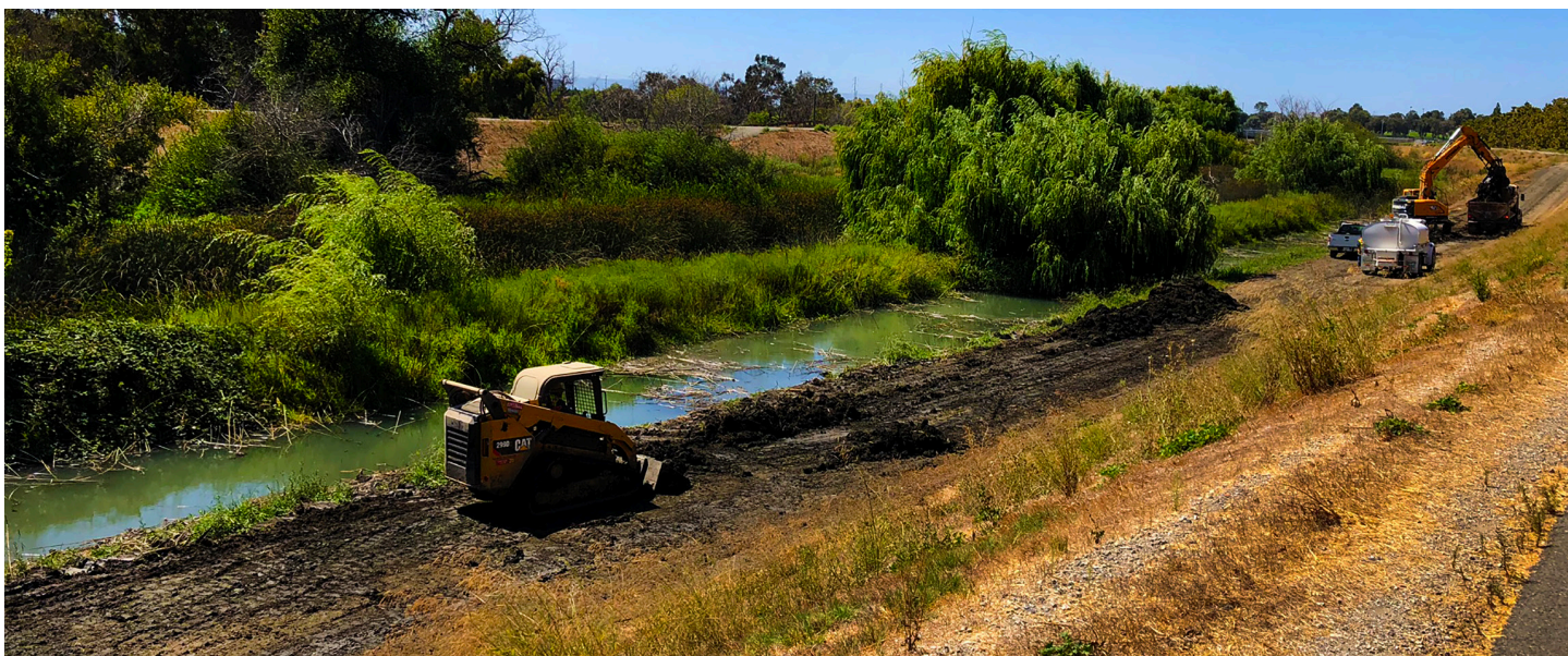
Valley Water maintenance work to remove sediment along the east bank of Guadalupe River, upstream of Tasman Drive.
