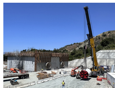
Diversion Outlet Structure nearly complete. Micro Tunnel Boring Machine assembly.
