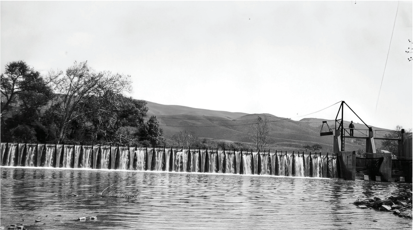
Figure 7. Historic view showing water flowing over the Coyote Percolation Dam's flashboard while a staff member oversaw crane operations. Photographer unknown, Coyote Percolation Dam, February 1, 1934 (on file at Valley Water's archives).
