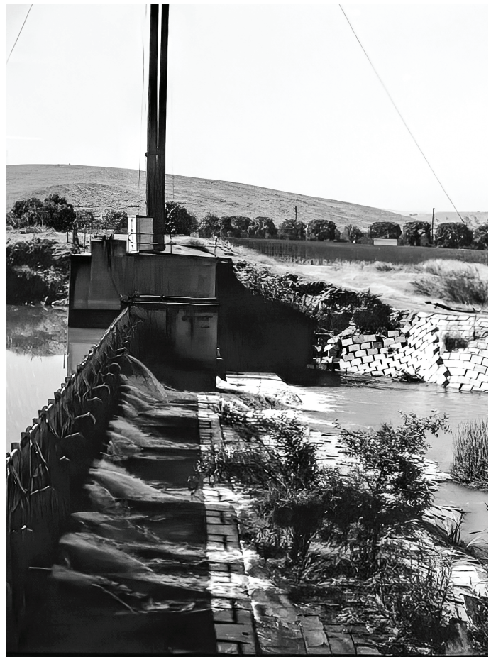
Figure 4. Historic view of the Coyote Percolation Dam. Photographer unknown. Coyote Percolation Dam, erosion of left bank [photograph], June 27, 1960 (photograph on file at Valley Water's archives).
