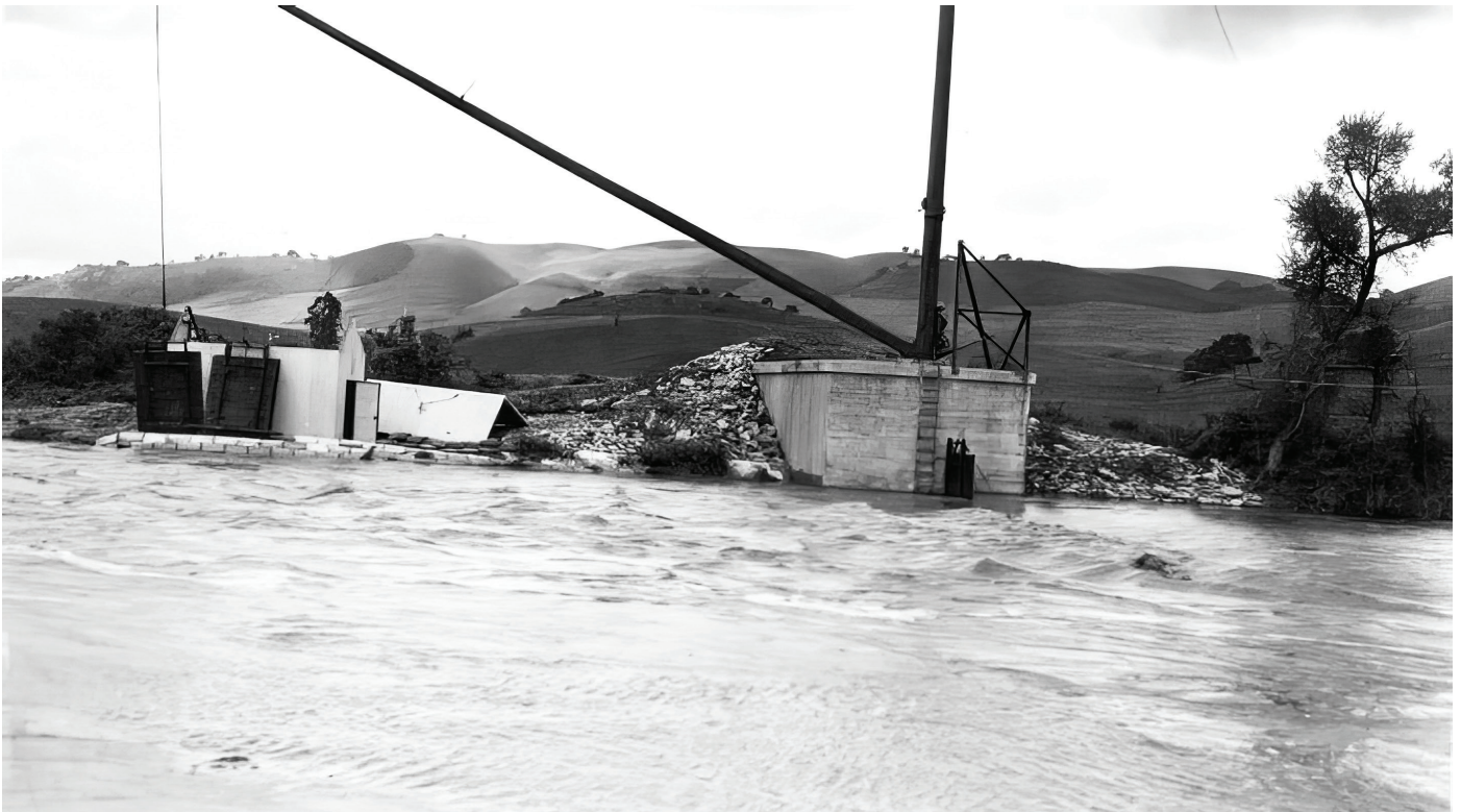
Figure 9. A derrick crane placed removed flashboard panels next to a utility building at the Coyote Percolation Dam. The removable gable roof appears to the right of that building. Photographer Unknown, Coyote Percolation Dam, April 8, 1935 (on file at Valley Water's archives).
