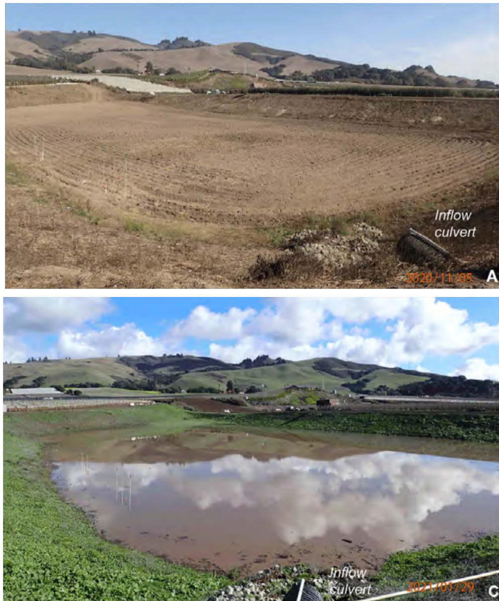
Figure II-1. Hillslope-runoff collection and infiltration project at Bokariza-Drobac Ranch, showing the 4.3 acre infiltration basin during dry conditions (top) and wet conditions (bottom). Photo credit: A. Fisher (UCSC).
