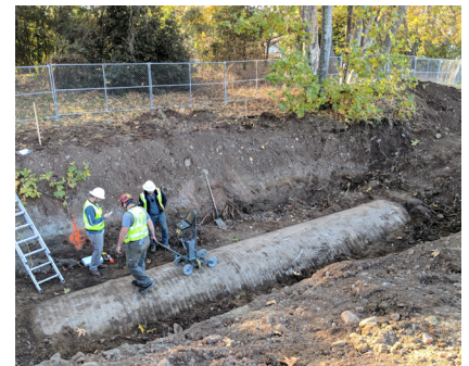
Inspection of Cross Valley and Calero Pipeline.
