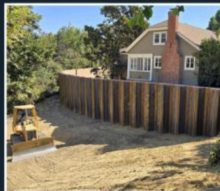
A floodwall was installed behind homes along S. 17th St.
