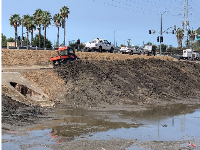
Beginning of Reach 8 at Confluence with Thompson
