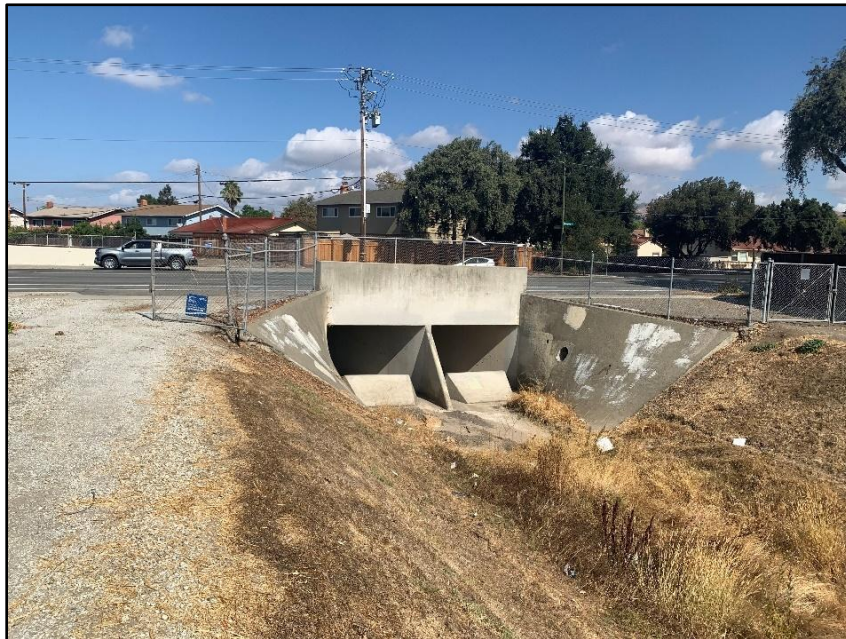
Reach 9 – Looking at Cropley Avenue culvert entrance
