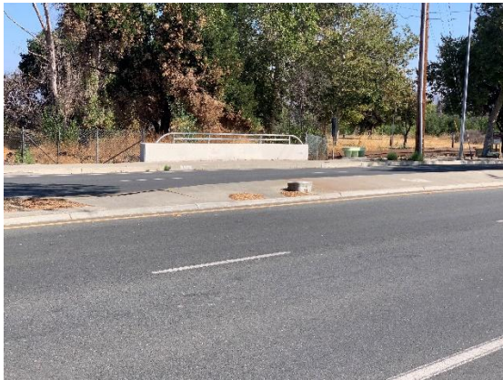
Looking upstream at upper Mabury Road crossing.
