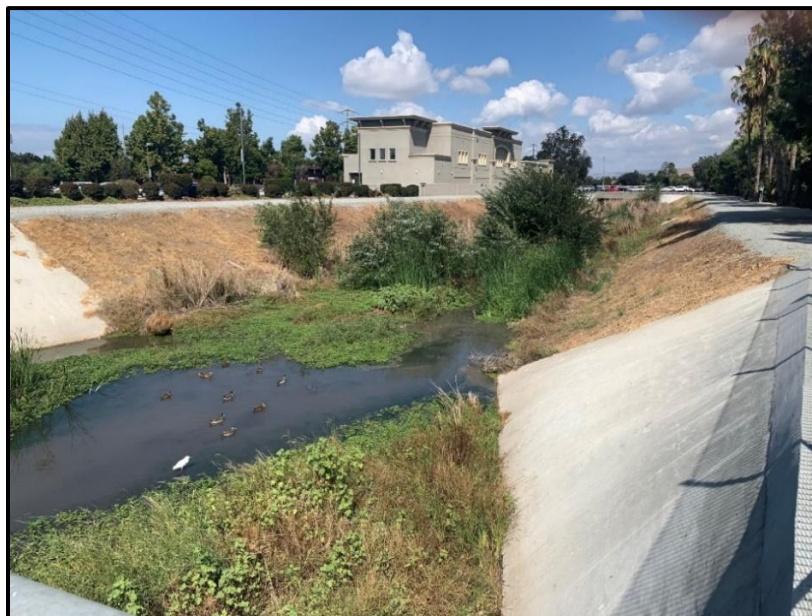
Reach 5 – Looking downstream from Los Coches Street toward Calaveras Boulevard
