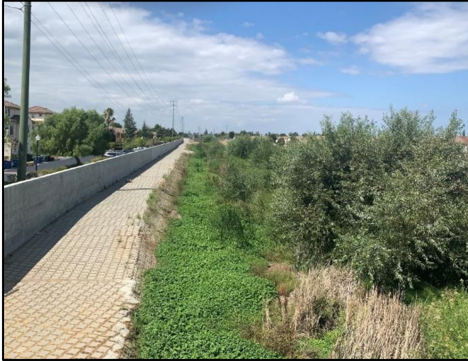
Reach 3 – Looking downstream from pedestrian bridge at south floodwall
