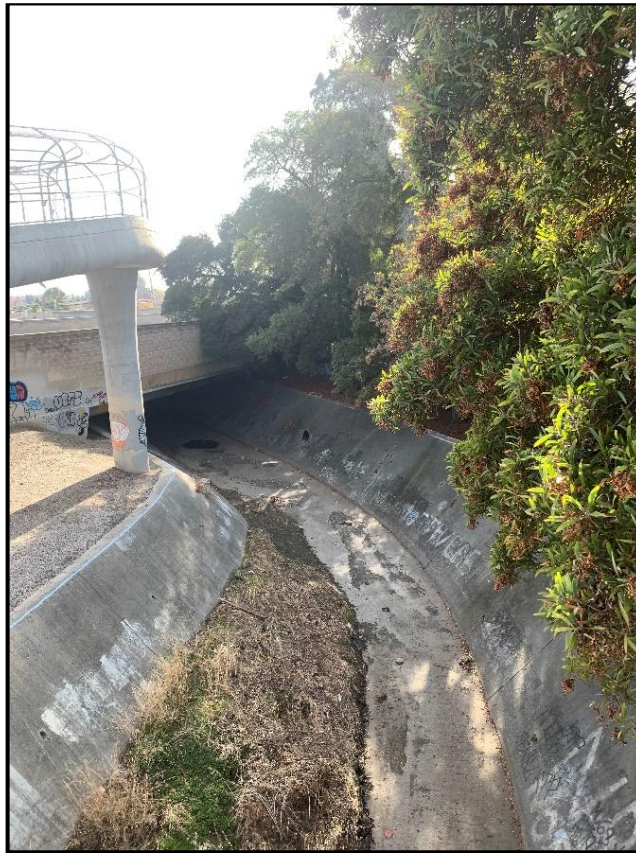
Reach 7 – Looking upstream at I-280 crossing
