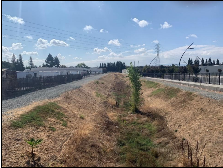
Reach 7 – Looking upstream from Montague Expressway
