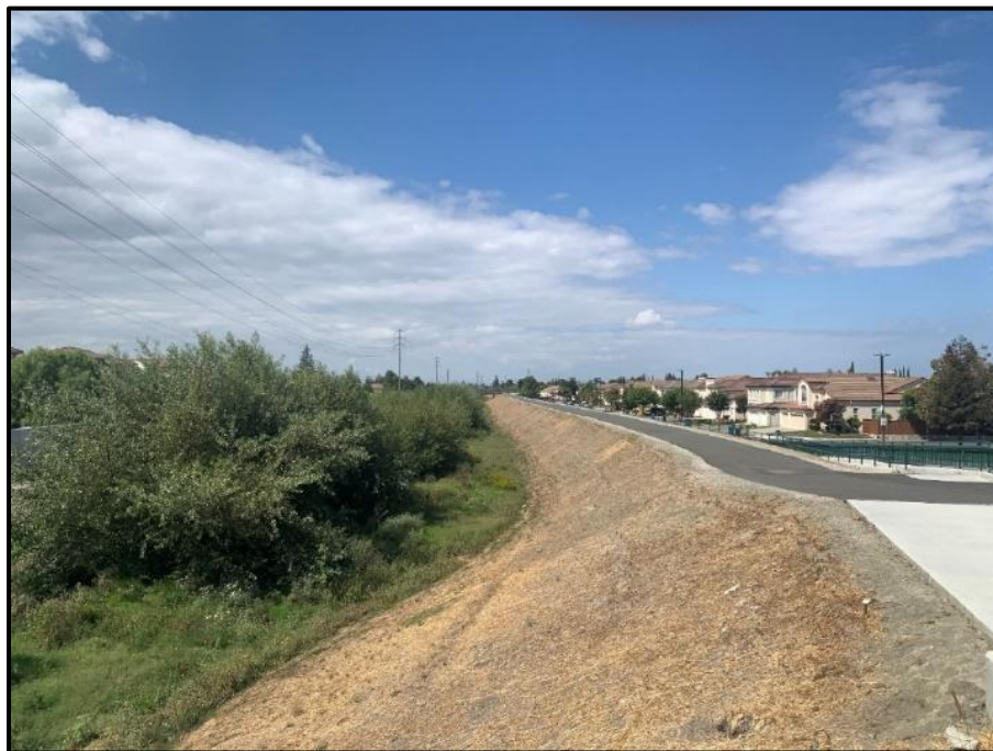
Reach 3 – Looking downstream from pedestrian bridge at north levee
