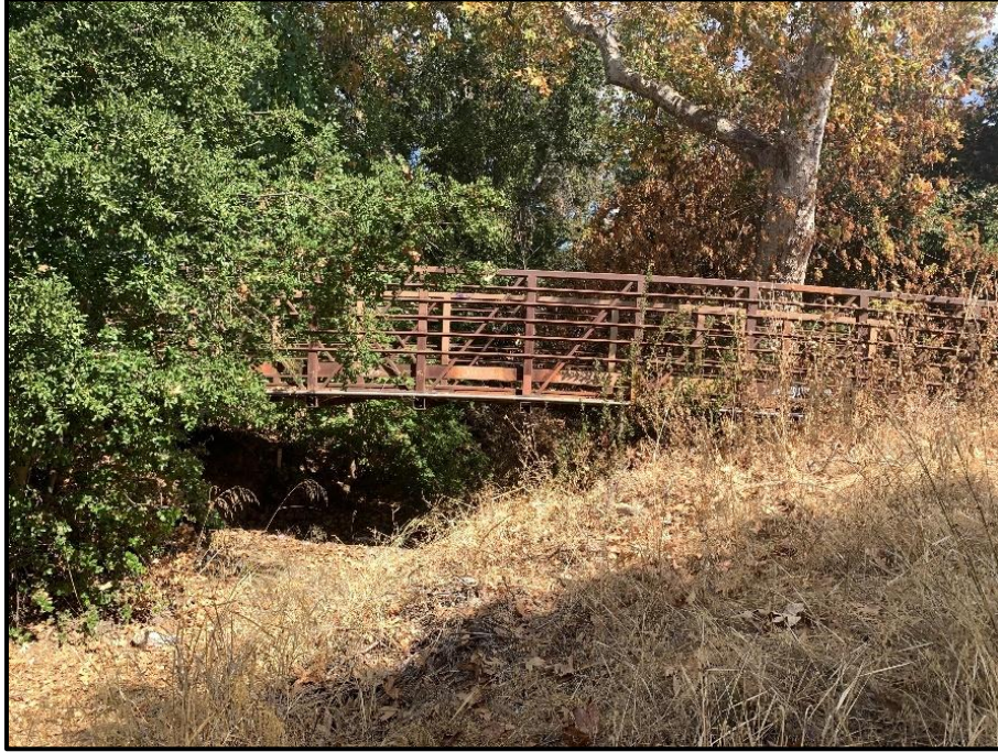
Reach 11 – Messina Drive pedestrian bridge
