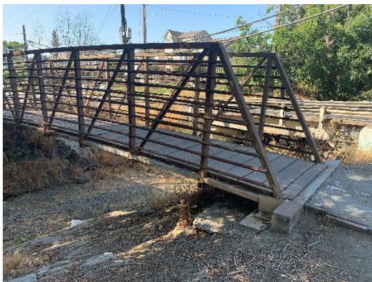
Looking downstream at King Road & Ped bridge
