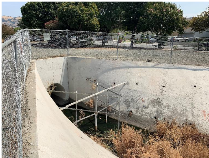
Upstream end of Reinforced Concrete Pipe at Mayfield Park
