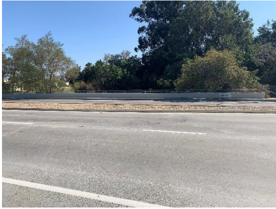
Looking upstream across Jackson Ave bridge.
