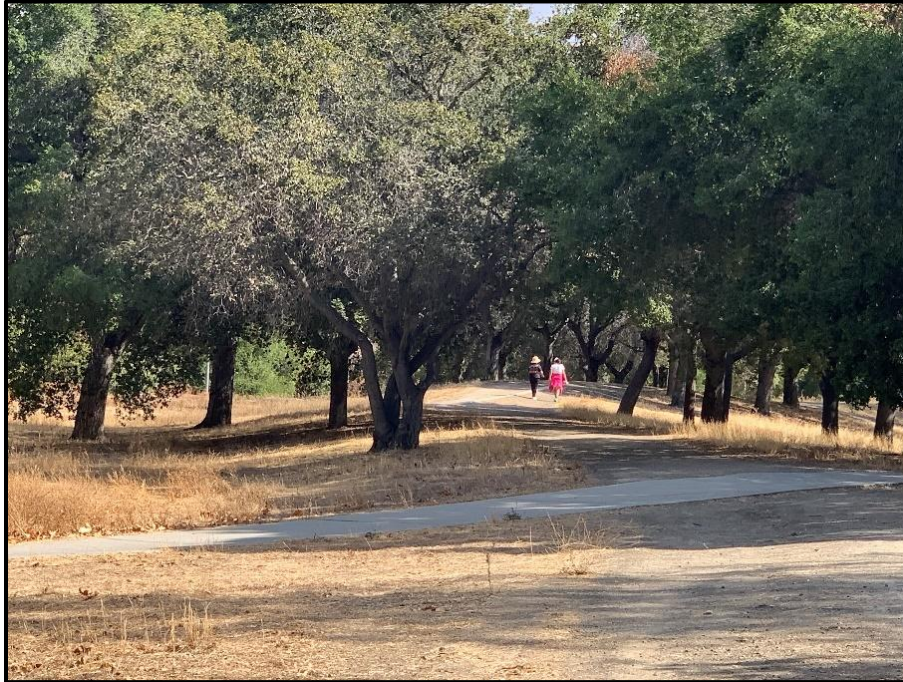
Reach 11 – Looking upstream of Messina Drive at the levee
