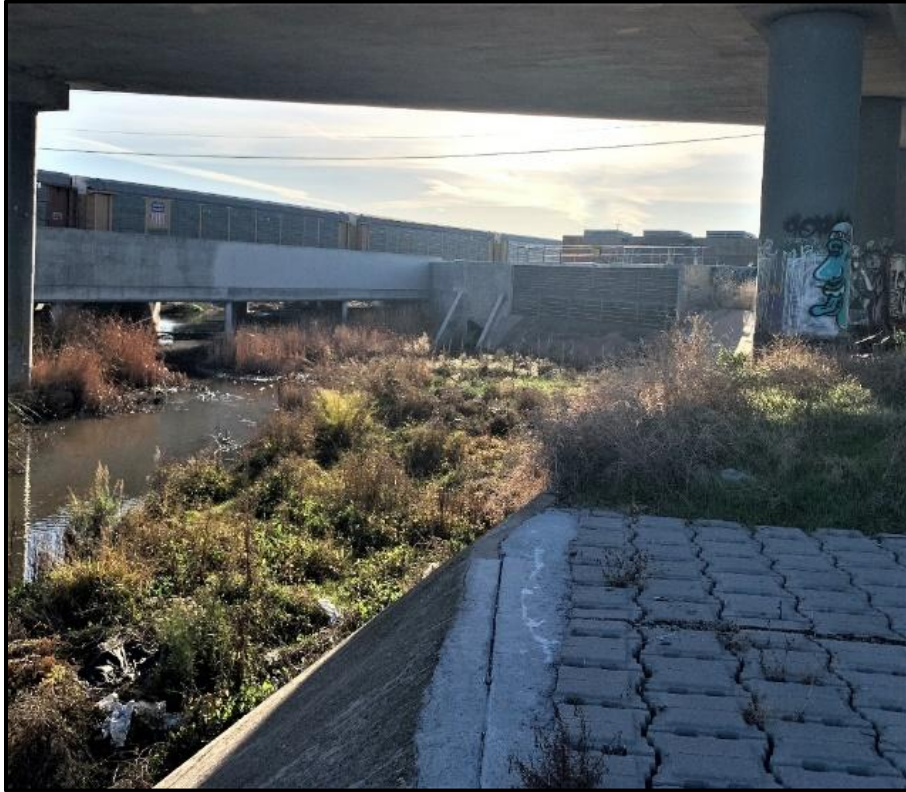
Reach 2 – Looking upstream from Abel Street at UPRR crossing and City of Milpitas Wrigley-Ford Creek Pump Station on right
