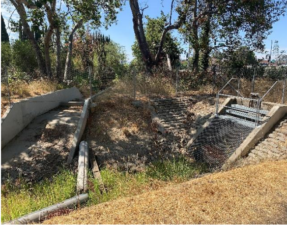
Pond overflow to creek near Piedmont Rd.
