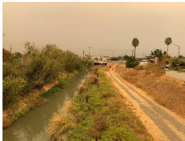
Looking downstream at the McKee Road culvert
