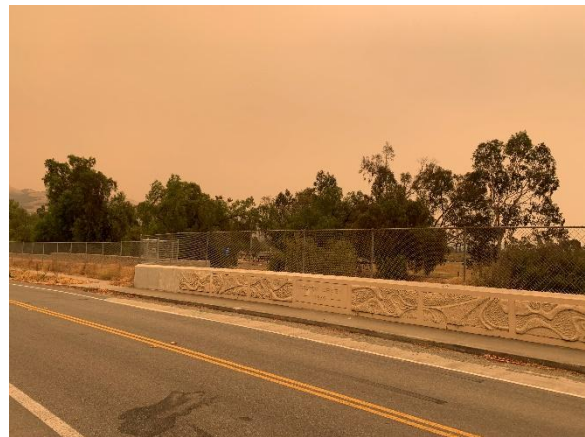
Looking south and east at Cunningham Avenue headwall and floodwall
