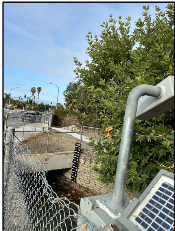
Reach 12 – Upstream Cropley Road entrance to the 400-foot culvert with visual gauge and web cam
