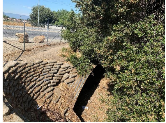
Upstream Jackson Ave culvert entrance.
