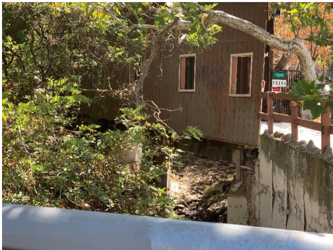
Just upstream Dorel Drive looking at a private bridge crossing.
