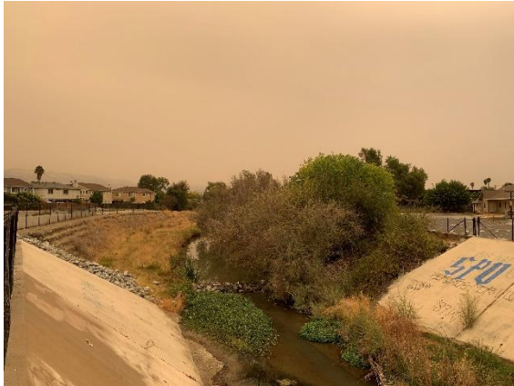
Looking upstream from San Antonio Road
