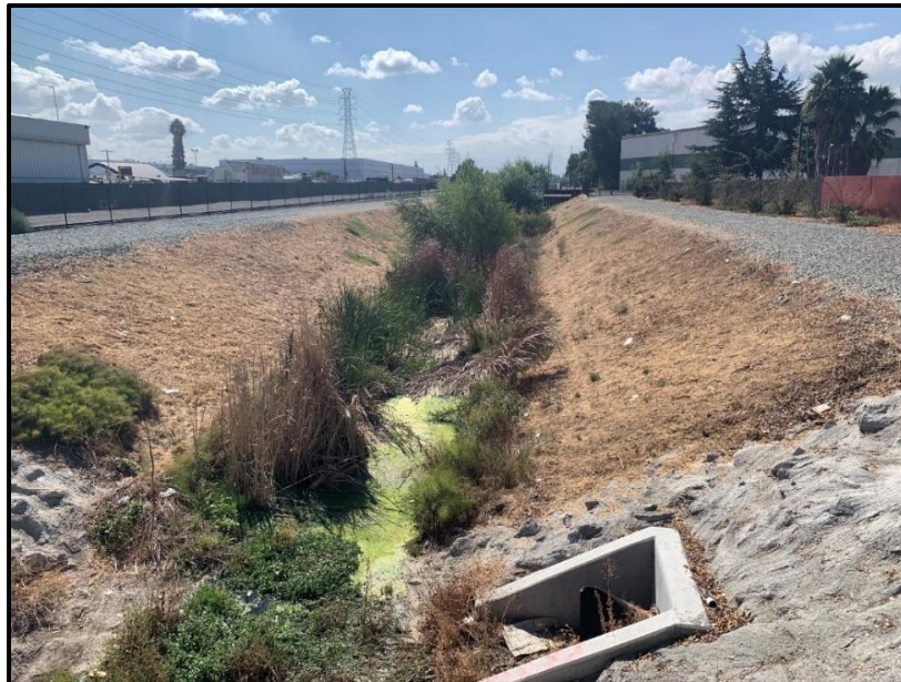
Reach 6 – Looking upstream from Yosemite Drive
