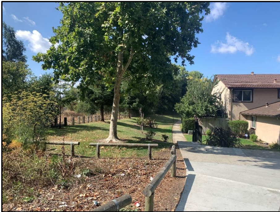
Reach 11 – Looking downstream of Messina Drive at levee on north side of creek
