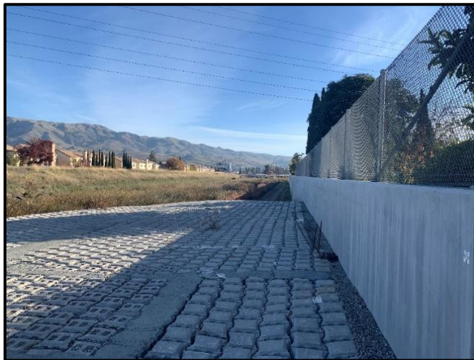
Reach 1 – Looking from Lower Penitencia Creek floodwall on right and levee on left
