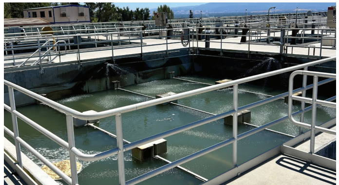
Flocculation and Sedimentation Basins
