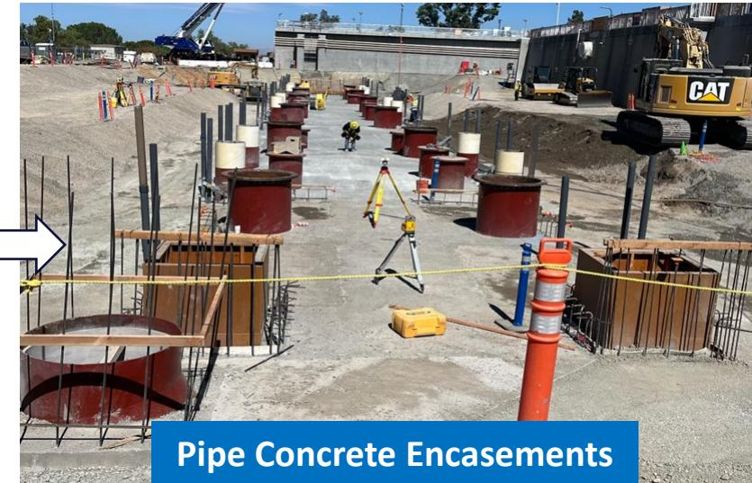
Pipe Concrete Encasements
