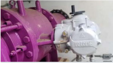
Plunger Valve at Main Avenue Ponds Vault.
