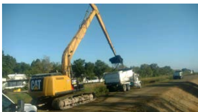
Sediment removal at Sunnyvale East Channel.
