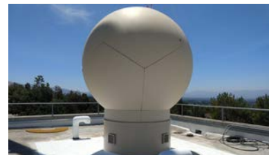
X-Band radar atop Penitencia Water Treatment Plant.
