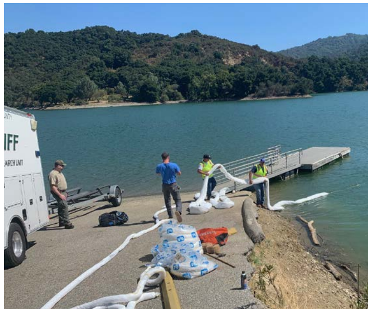
Boom deployment at Stevens Creek Reservoir.
