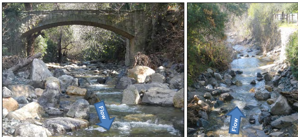
Figure 2-3 Chutes-and-Pools Roughened Channel on an Incised Reach of Penitencia Creek in Alum Rock Park, San Jose, California
