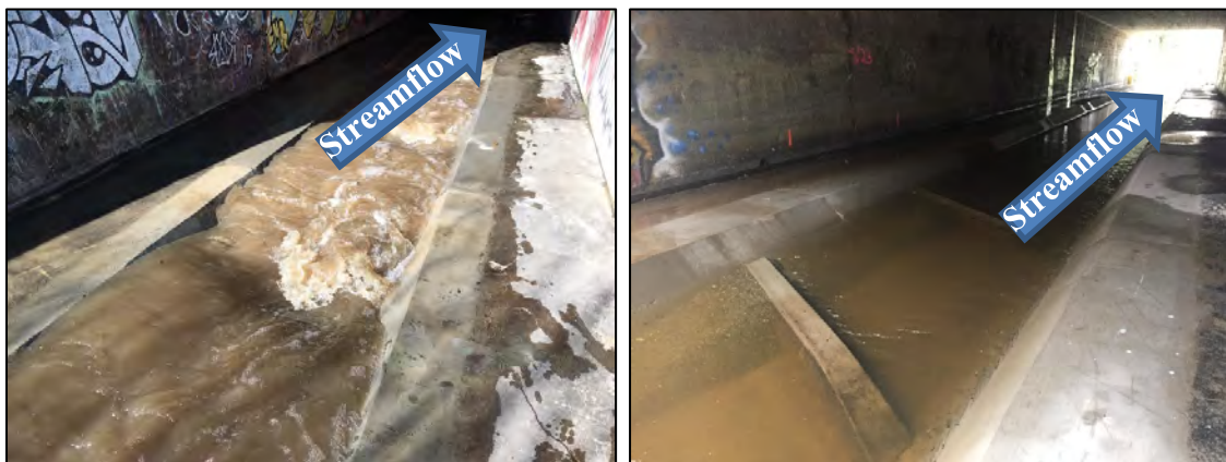
Figure 2-6 Fish Transport Channels (Looking Downstream), with Notches and Fish Baffles to Control Depths and Velocities under Interstate 80 on Pinole Creek in Pinole, CA (left image) and on Strongs Creek in Fortuna, CA (right image)
