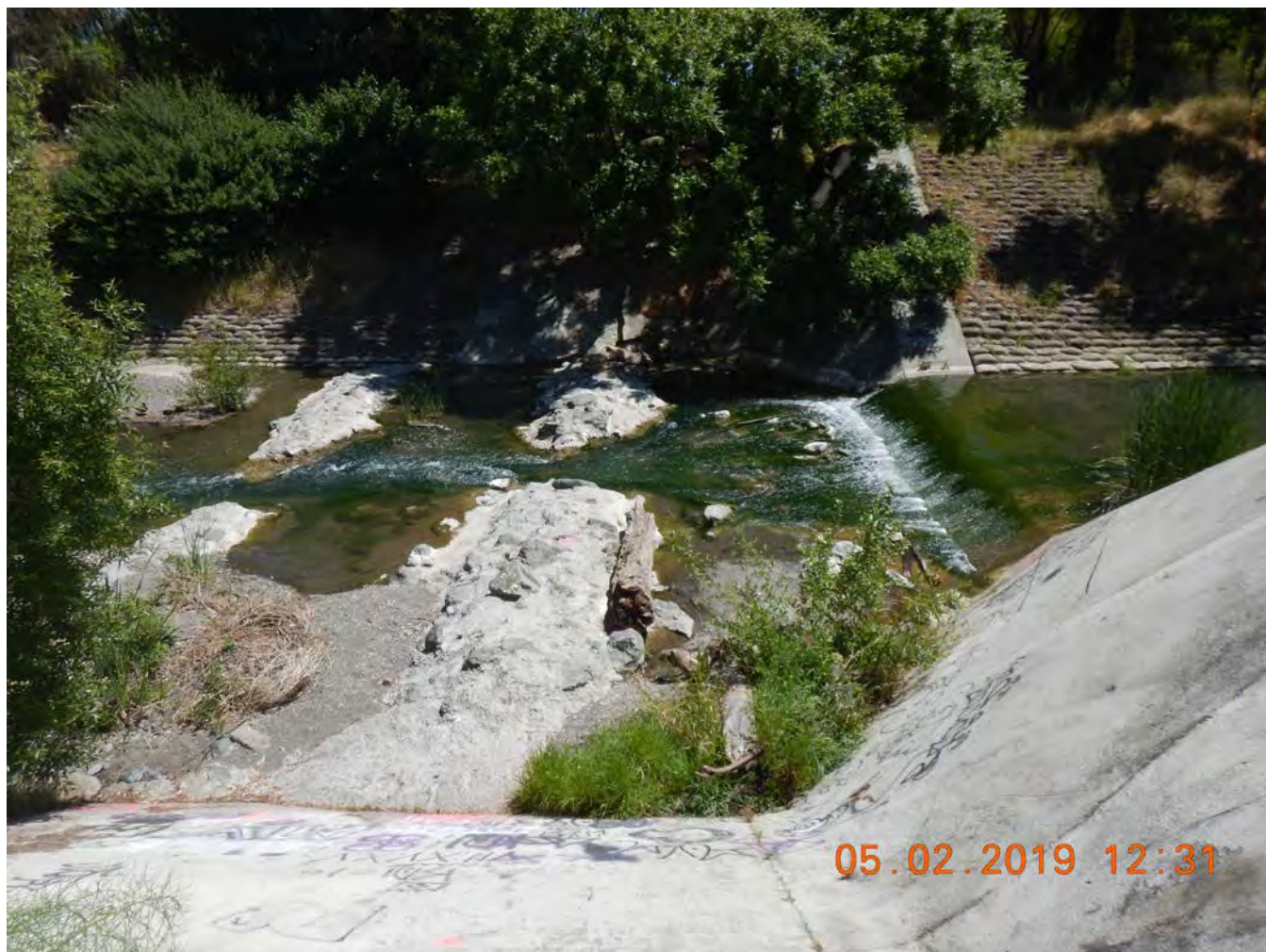
Photograph 4: Grade control structure at Vernon Avenue
