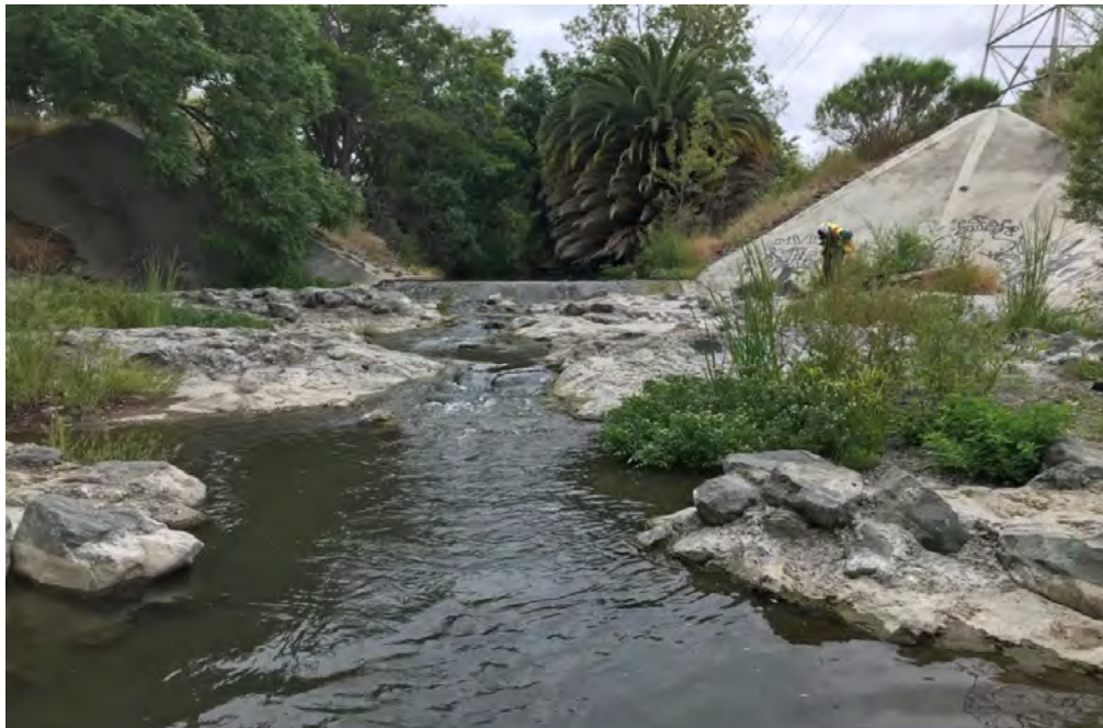
View from downstream looking upstream at grouted rock veins and concrete drop structure
