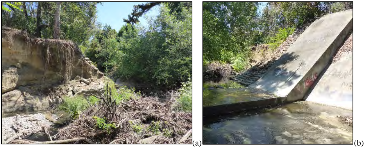
Figure 3-2 Site 9 – Looking (a) Downstream, Where the Stream Flows Directly into a Failing Bank before Turning Right and Going Over the Site 9 Drop Structure, and (b) Looking Upstream at Site 9, with Failing Banks in Background
