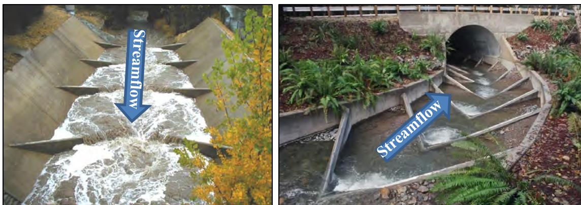
Figure 2-5 Vortex Pool-and-Chute Fishway on Stevens Creek at Gage SF35 (left image) and in Del Norte County, California (right image)
