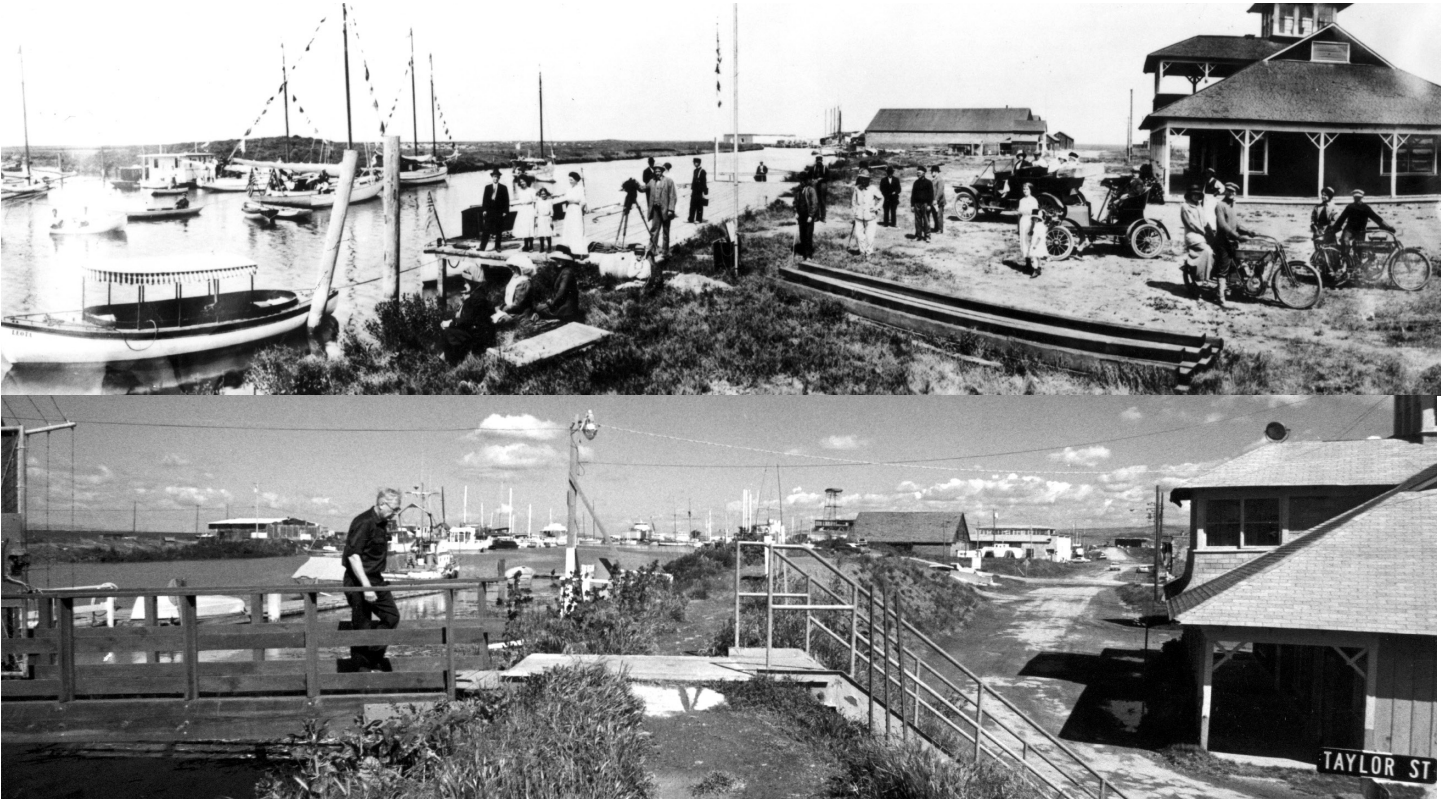
Levees prevent bay flooding at the Alviso Marina where the land sank more than six feet from subsidence between the early 20th century (top photo) and 1970s (bottom photo).
