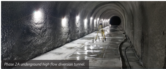
Phase 2A underground high flow diversion tunnel.
