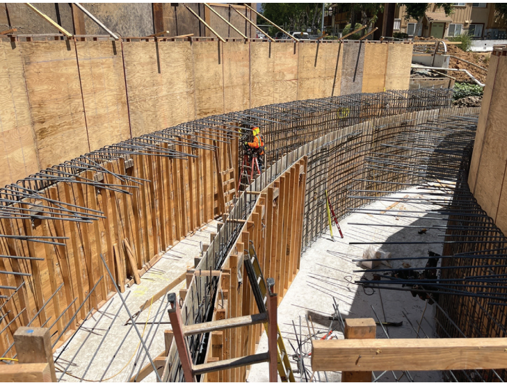
Phase 2A underground twin reinforced box culvert construction completed in 2024 at Hale Avenue and W. Main Avenue in Morgan Hill.
