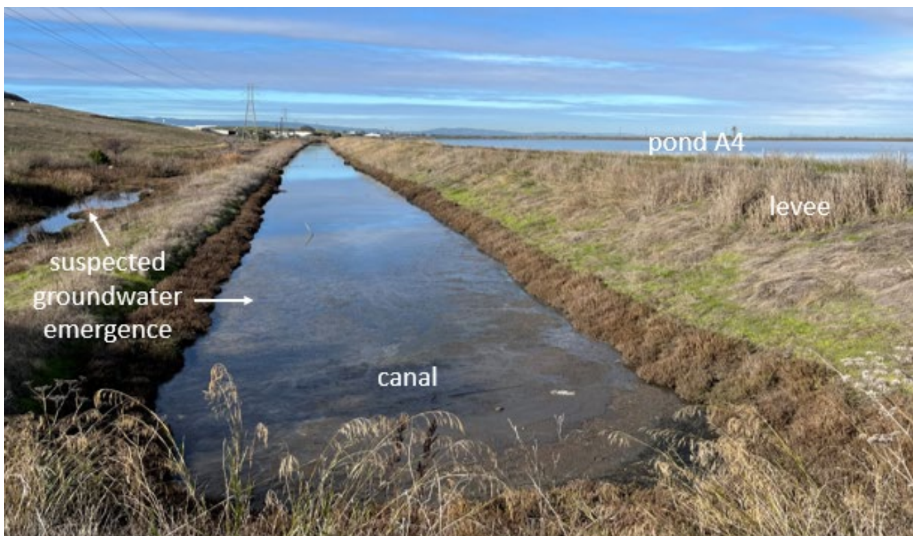
Figure D-20. Suspected groundwater emergence at the canal on the north side of Location 4 during the 2024 king tide events
