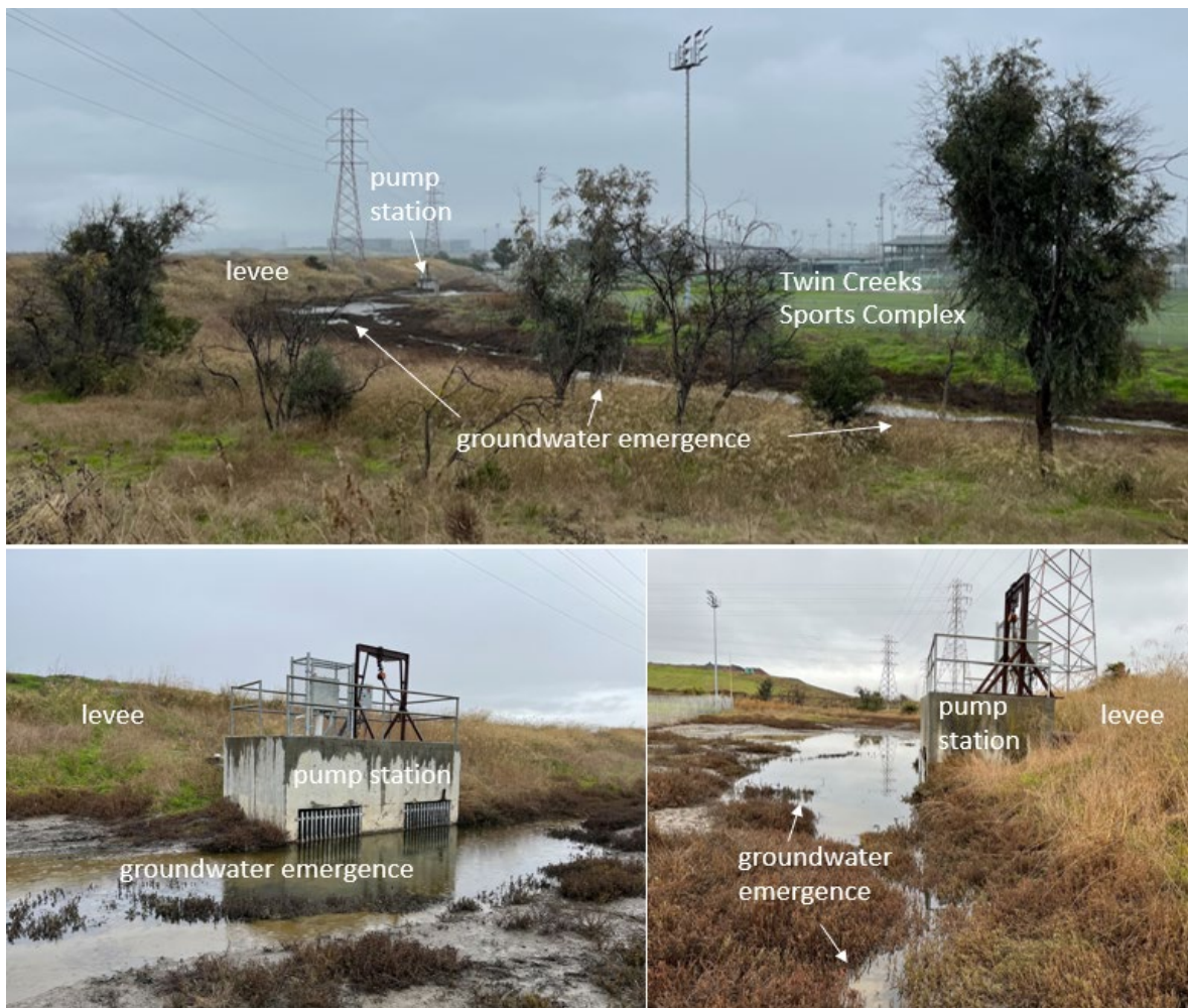
Figure D-17. Groundwater emergence northwest of Twin Creeks Sport Complex in Location 4 during the 2024 king tide events
