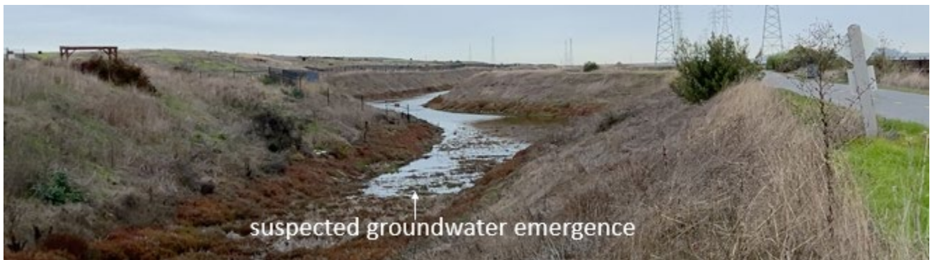
Figure D-13. Suspected groundwater emergence at the canal area in Location 2 during the 2024 king tide events
