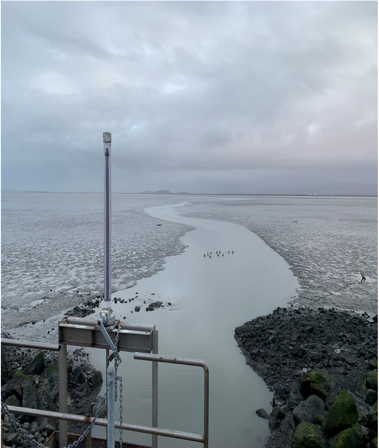
Tide gate on the Bay side of salt ponds AB1 and AB2 during low tide, exposing a channel in the Bay Mud that has formed from water flowing in and out through the tide gate. Photo credit: Scott Elkins, Valley Water, taken September 16, 2024 during a spring tide (see Chapter 3).
