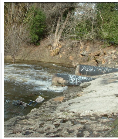
Photo 1: Singleton Road Fish Passage Barrier
