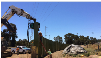
Sheet pile installation work.
