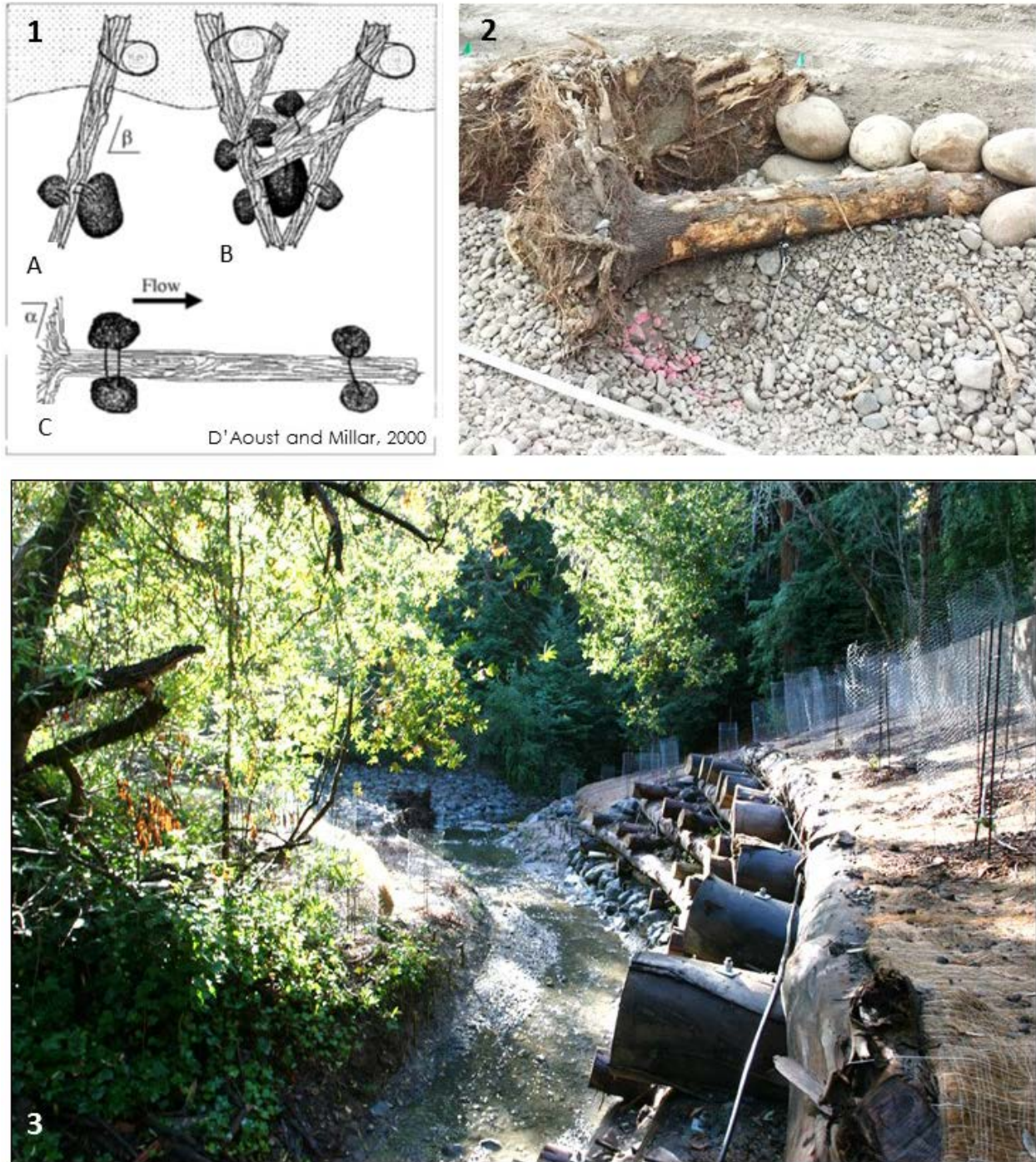
Figure 4-3 Examples of stabilizing methods for large woody debris. Panel 1 illustrates methods for ballasting logs, and engineered log jams with large boulders. In addition, Panel 1 illustrates pinning large woody debris to living trees on streambanks. Panel 2 illustrates a rootwad placement which utilizes ballast/burial in tandem with cabling. Panel 3 illustrates a bio-engineered cribwall.
