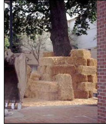
Photo 5: Stacked hay bales protect trunks from damage from incidental contact.
